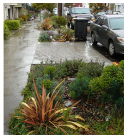
Planters and permeable pavers can be used to reduce stormwater impacts.
