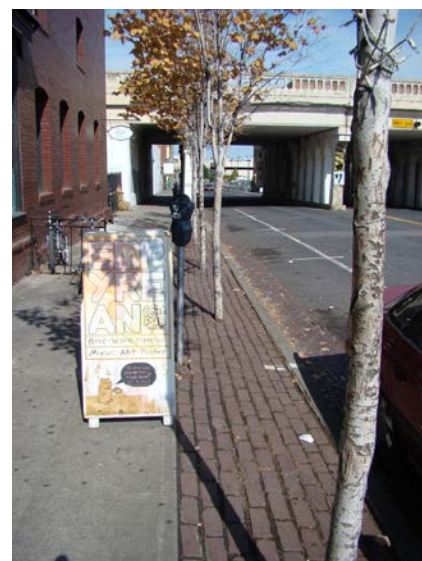
Permeable paving helps reduce impervious surfaces in pedestrian walkways.
