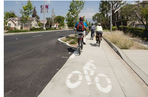
Separated and dedicated bike facilities that provide separation from motor vehicles.
