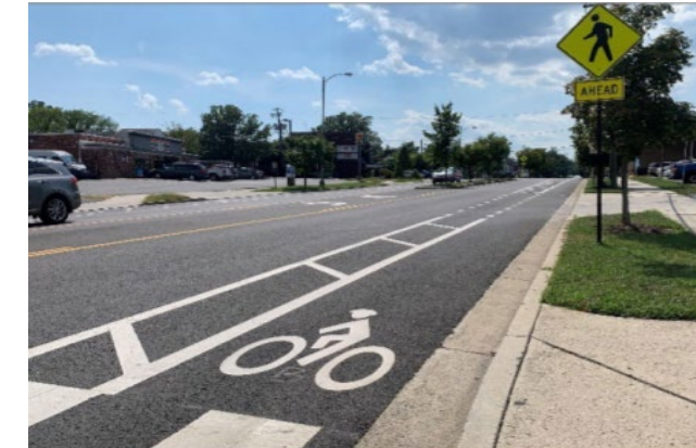
Buffered bike facilities that provide increased separation from motor vehicles with pavement markings.
