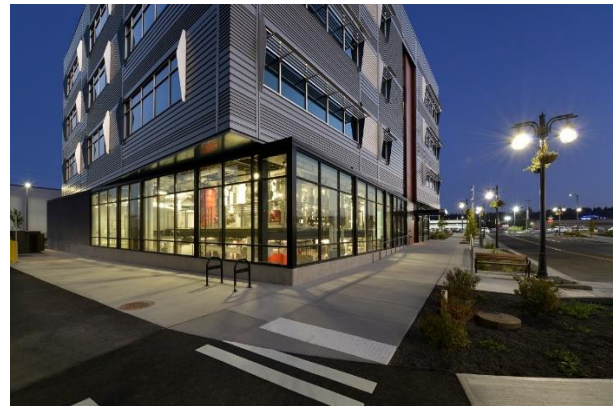
Figure 40. Morris Center Office Building (Built 2020)
