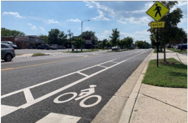
Buffered bike facilities that provide increased separation from motor vehicles with pavement markings.
