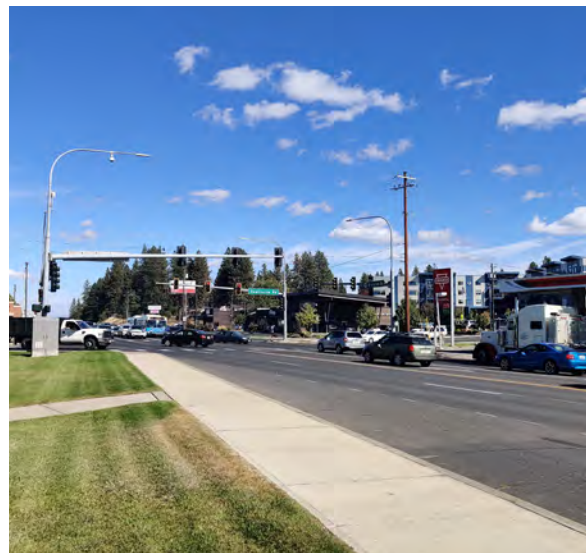
Figure 2. Existing Division Street Corridor
