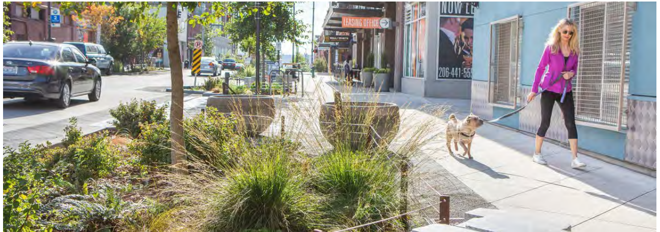
Figure 73. Stormwater bioswale along sidewalks increase stormwater management
