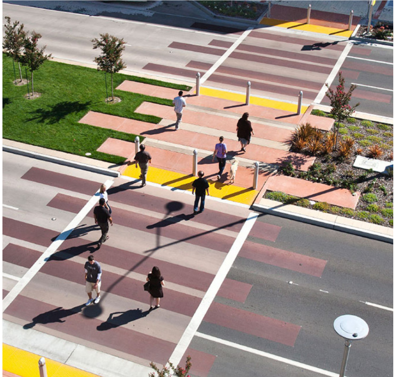
Figure 58. High-visibility crosswalks increase mobility across multiple lanes of traffic or high-traffic areas
