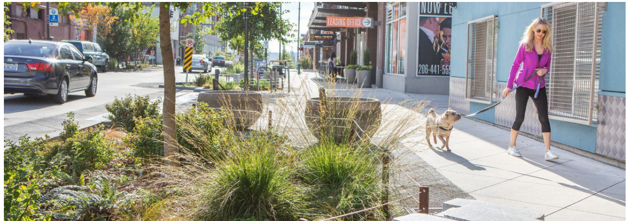
Figure 73. Stormwater bioswale along sidewalks increase stormwater management
