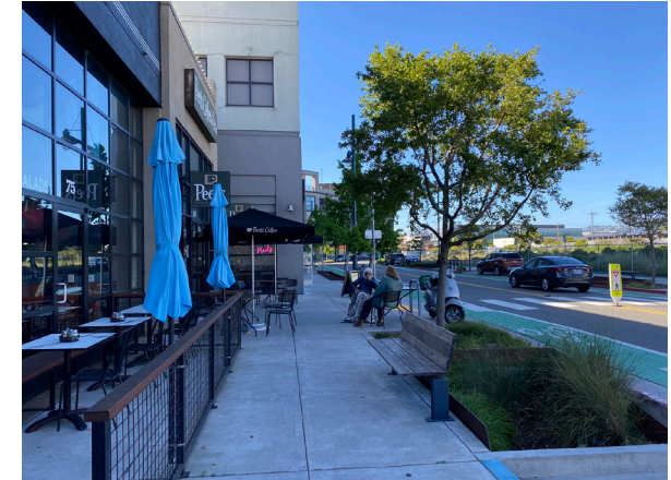
Figure 27. Building front setbacks allow for more sidewalk activation
