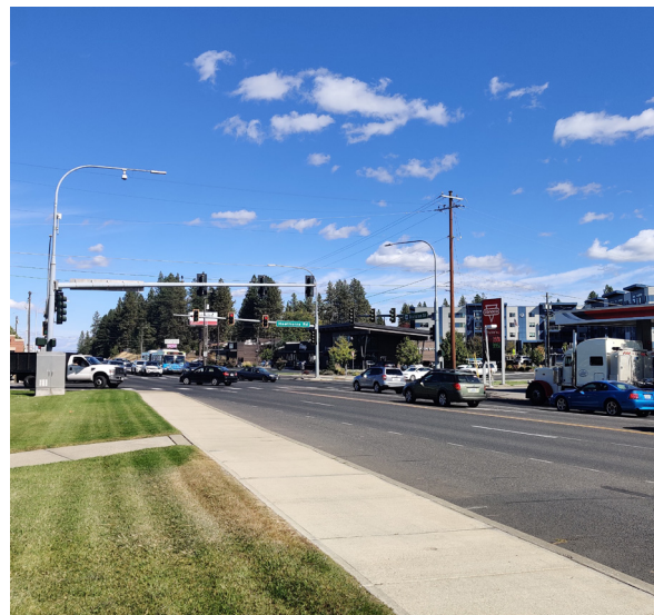
Figure 2. Existing Division Street Corridor
