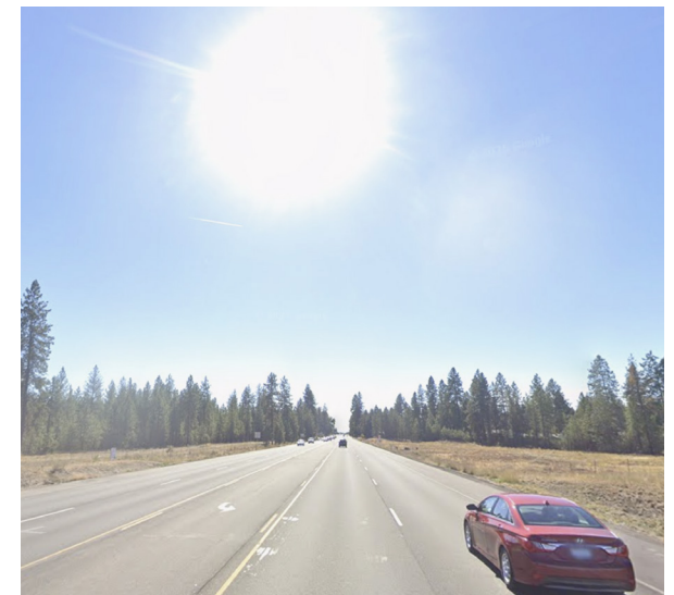
Figure 199. Sparse sidewalks reduce connectivity
