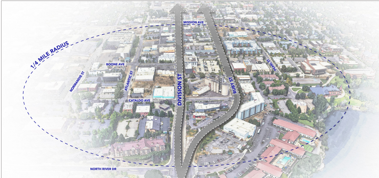
Figure 127. Existing aerial view of South Couplet
