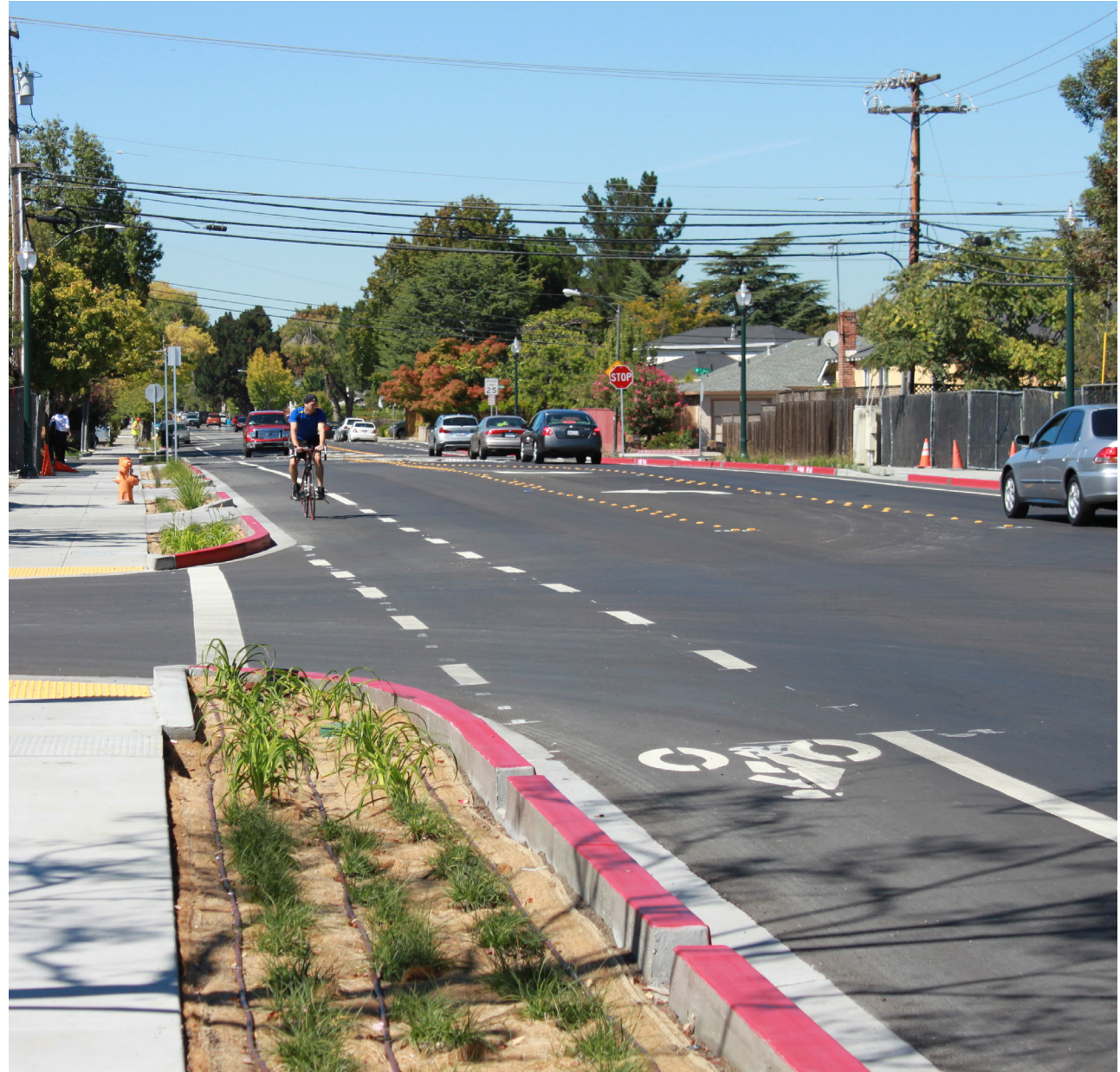
Figure 51. Bike facilities along a lower-speed neighborhood connector street can increase comfort for those biking
