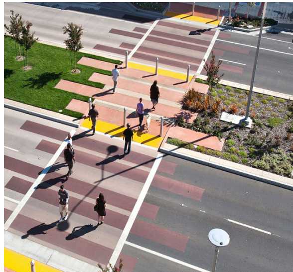
Figure 186. Enhanced crossing provides a buffer between vehicles and pedestrians
