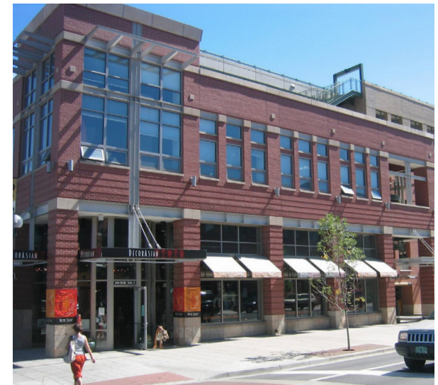
Figure 32. Building entrances with weather protection allow people access year-round
