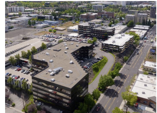
Figure 118. Rock Pointe employment area shows different building heights and transitions
