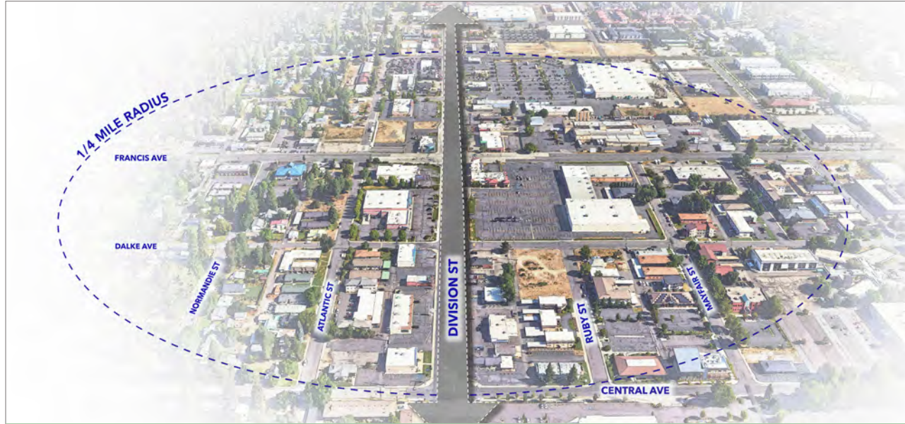
Figure 171. Existing aerial view of Francis/Lyons
