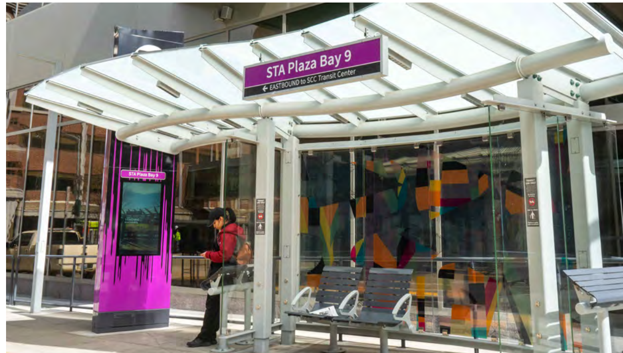
Figure 91. The STA has been implementing station areas successfully
