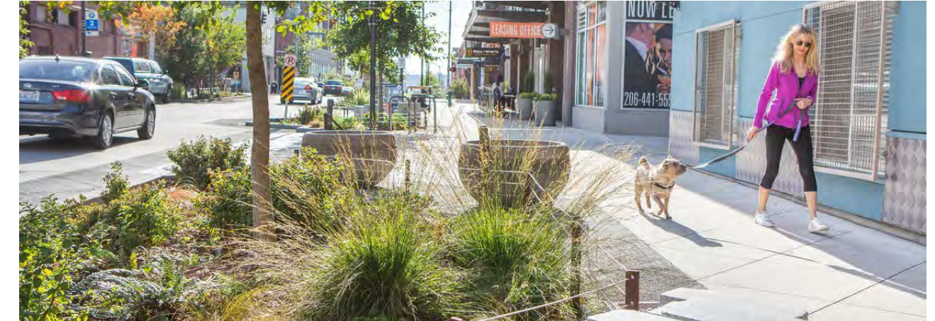
Figure 73. Stormwater bioswale along sidewalks increase stormwater management
