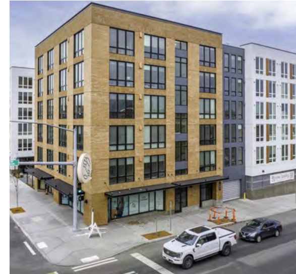
Figure 12. Podium Style Apartments in Downtown Spokane (The Warren)
