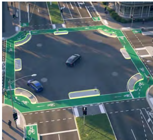
Figure 121. Enhanced crossing for bicycles can reduce conflict between cars and those biking
