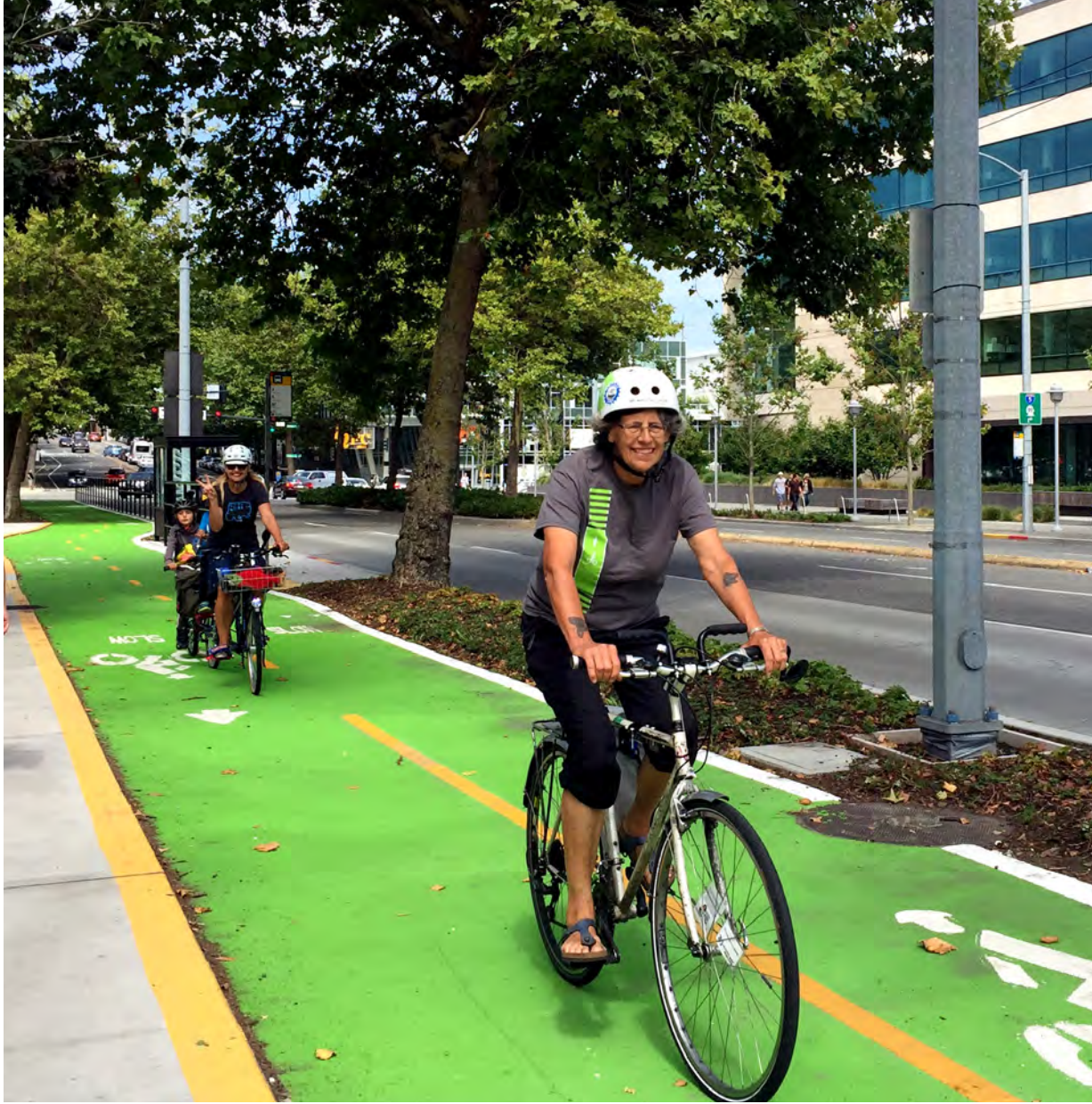
Figure 98. Designated bike lanes can help reduce the Bike Level of Stress (BLOS)
