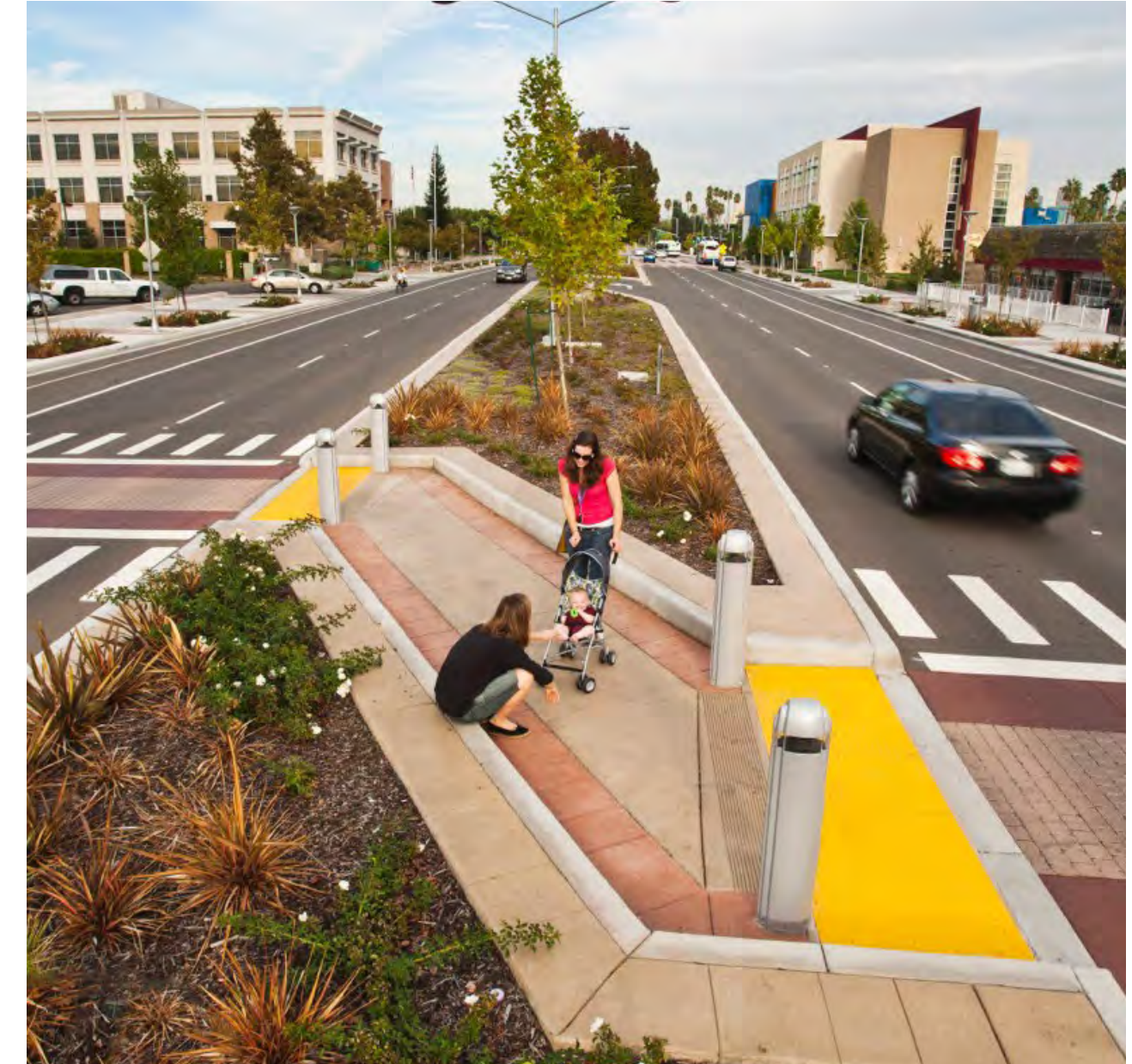
Figure 36. Mid-block crossing enhancements, like medians, allow for people to cross comfortably across multiple lanes of traffic
