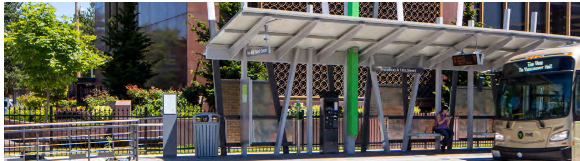
Figure 49. Bus Rapid Transit (BRT) amenities provide additional comfort for those using services
