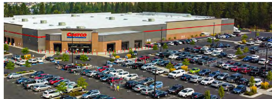
Figure 197. Costco is a major anchor within the node
