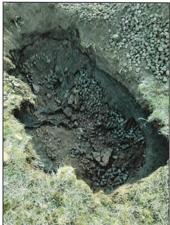
PHOTO 2: GEOFABRIC WITHIN TP-1
