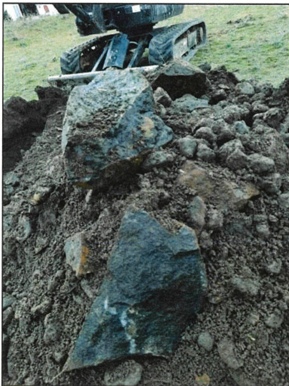
PHOTO 7: TP-2 EXCAVATED SOILS AND BOULDERS
