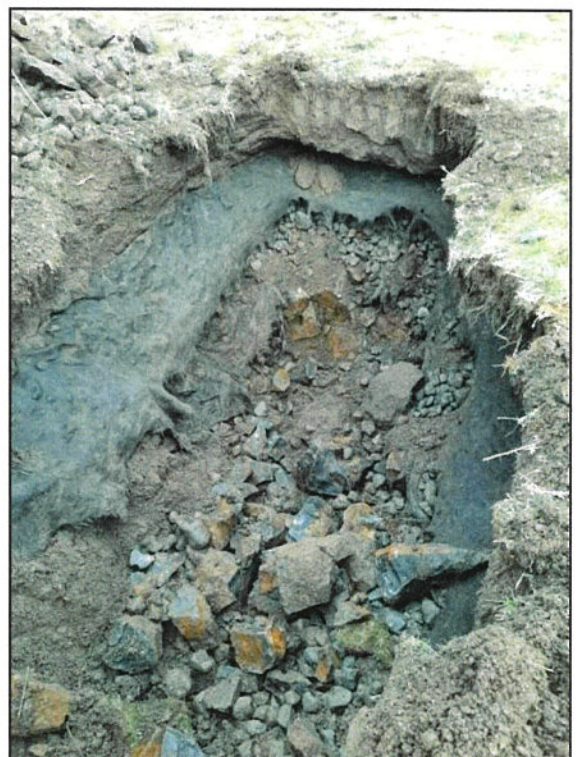
PHOTO 8: GEOFABRIC WITHIN TP-2
