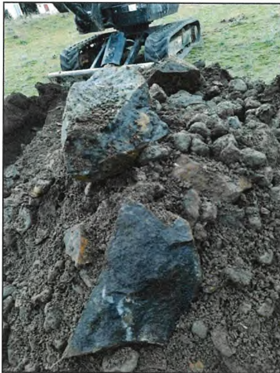
PHOTO 7: TP-2 EXCAVATED SOILS AND BOULDERS
