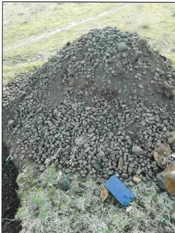
PHOTO 3: TP-1 EXCAVATED SOILS
