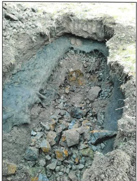
PHOTO 8: GEOFABRIC WITHIN TP-2
