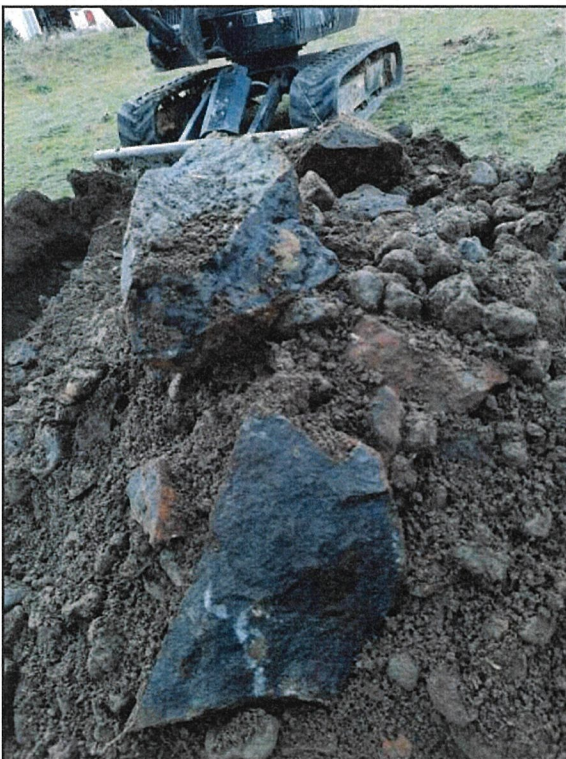
PHOTO 7: TP-2 EXCAVATED SOILS AND BOULDERS
