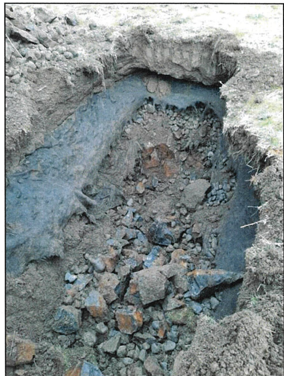
PHOTO 8: GEOFABRIC WITHIN TP-2
