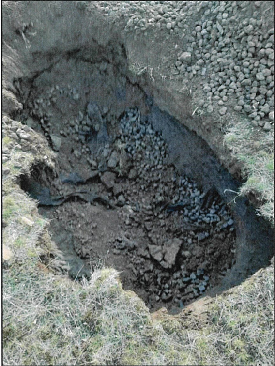
PHOTO 2: GEOFABRIC WITHIN TP-1
