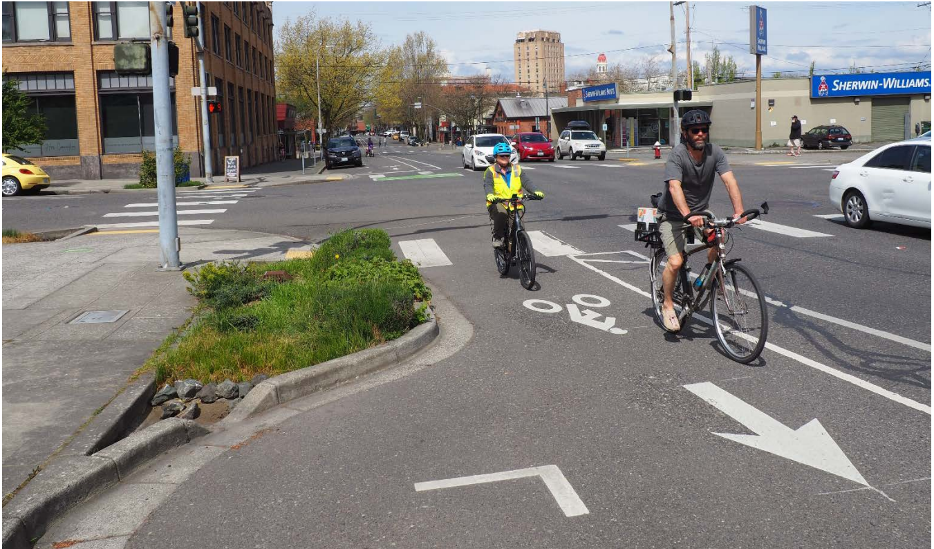
Figure 11: Example of a curb extension with green stormwater infrastructure in Bellingham, WA
