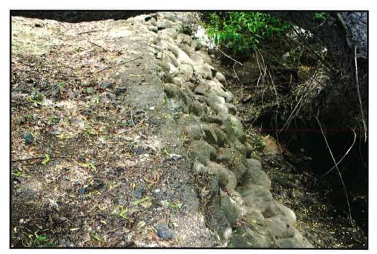
Figure 11. Mortared cobble and concrete retaining wall at site 45SP495, view to the north.
