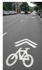
to remind all roadway users to share the road while directing cyclists out of the "door zone." On roads with steep terrain, a "climbing lane" should be used on the uphill side of the roadway and sharrows should be used to guide cyclists in the downhill lane.
