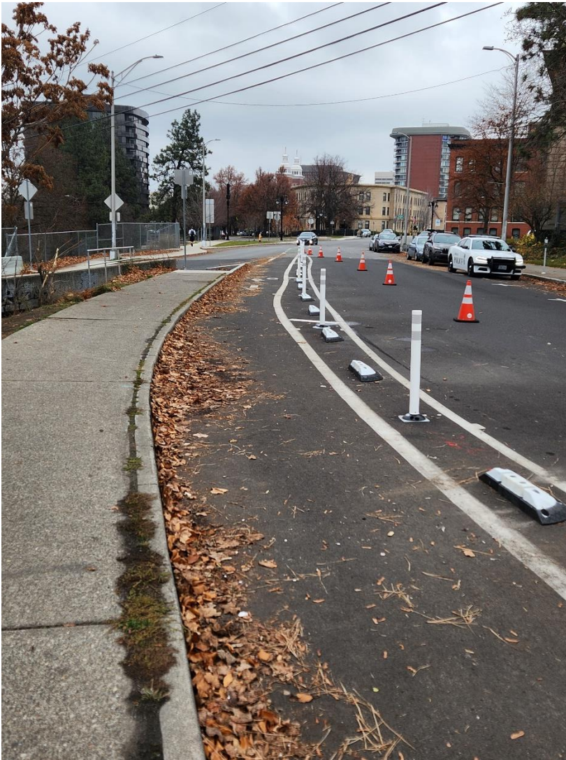
Photo: New bike lane hardening with Zicla Zipper System
