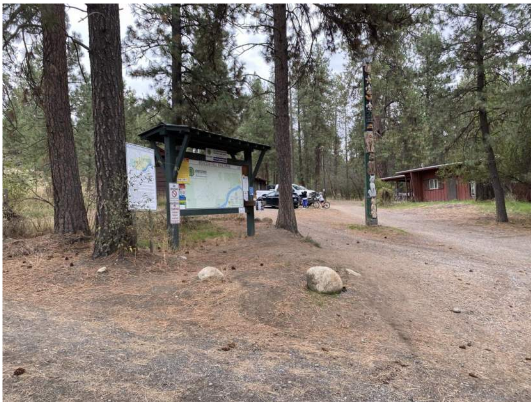
Photo 10. View of the existing structures within Camp Sekani. The building visible to the right will be demolished as part of the Proposed Project Action.
