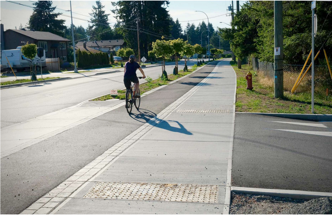
An example of a continuous sidewalk with a bike lane in Nanaimo, British Columbia, Canada taken by Roy Symons
