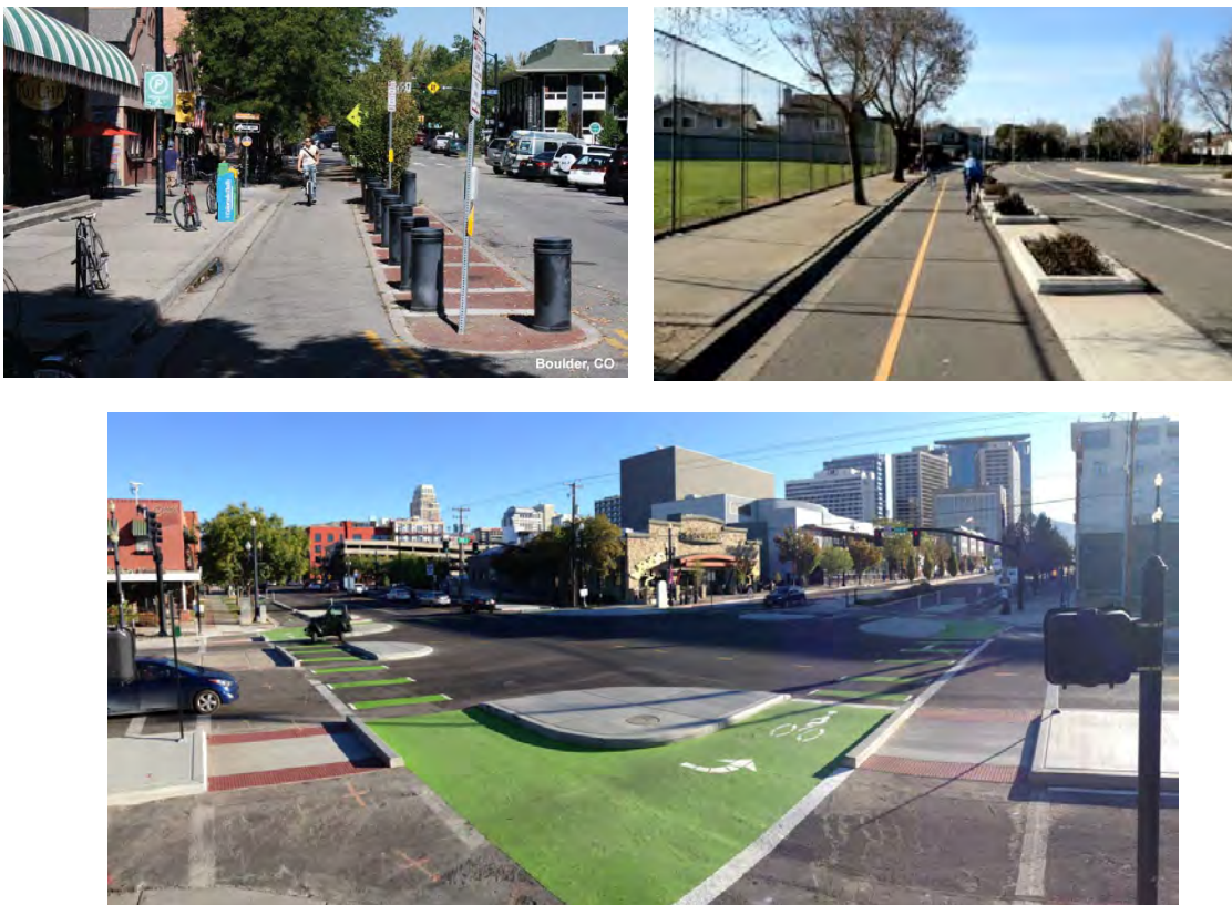
Figure 5. Examples of potential cycle-track protected bike lane designs
