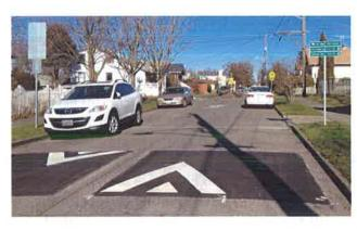
Figure D14 – Example of speed humps on a residential street in Spattle
