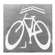
Figure D13 – A typical sharrow pavement marking.
