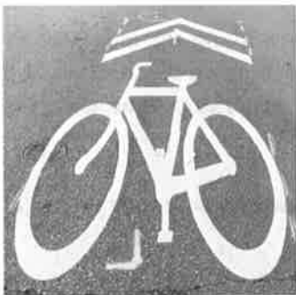
Figure D13 – A typical sharrow pavement marking.
