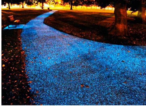
Figure 5.4.1 A StarPath – A coating that absorbs and stores UV rays during the day and then releases them at night, allowing particles to glow in the dark.
