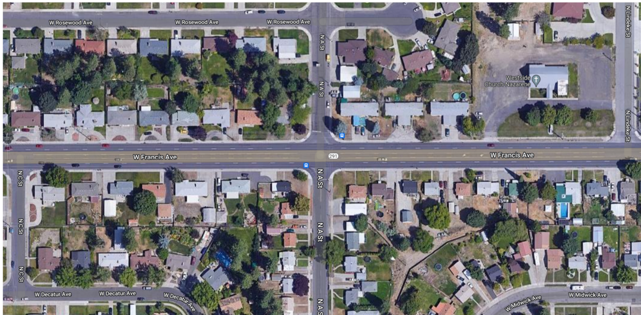
Francis Avenue and North A Street Intersection
