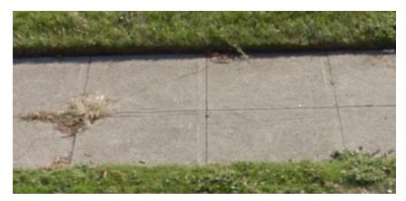
**<u>Cosmetic</u>**: A Cosmetic sidewalk will have insignificant cracking and weathering typical for outdoor concrete pours. Cosmetic sidewalk repairs will not be considered for replacement under this program.
