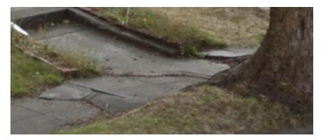
**Dangerous**: Sidewalks considered dangerous will have a lift greater than half an inch, significant cracking with widths exceeding one half an inch and significant deterioration making pedestrian access difficult. Only dangerous sidewalks will be considered for this program.
