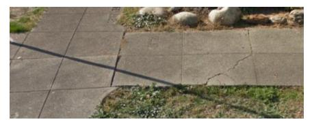
**Poor**: A sidewalk in Poor condition will have minor cracking and lifting not to exceed one half inch. Pedestrian access is not limited by a sidewalk in poor condition. Sidewalks in poor condition will be considered for replacement on a case-by-case basis, please avoid selecting sidewalks in poor condition.
