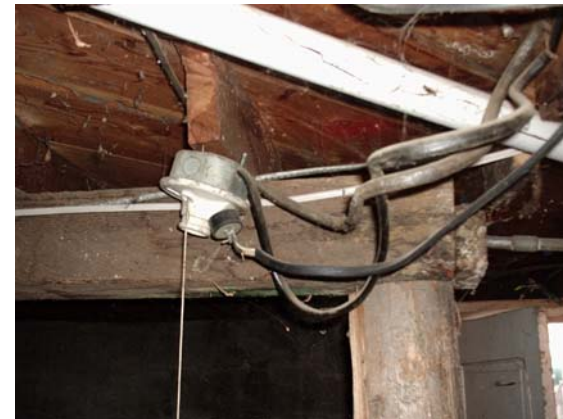
Hazardous Wiring, Altered Structural Member
