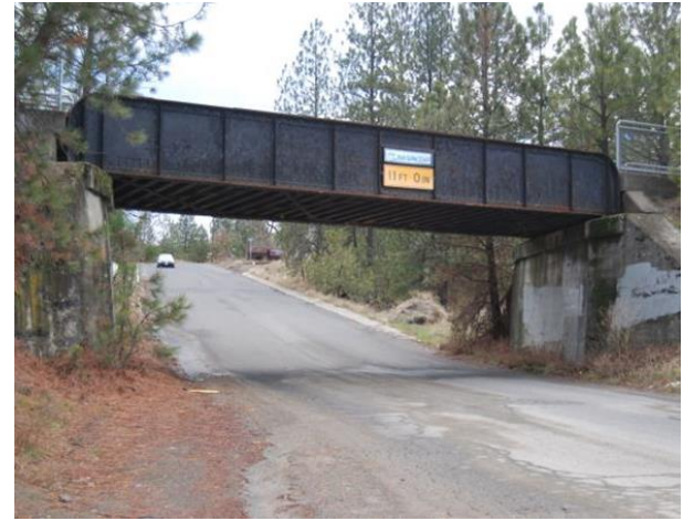
Photo: railway bridge above a street in Grandview/Thorpe
