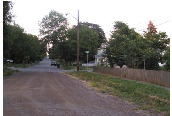
Unpaved section of North Hogan and Cataldo Street.
