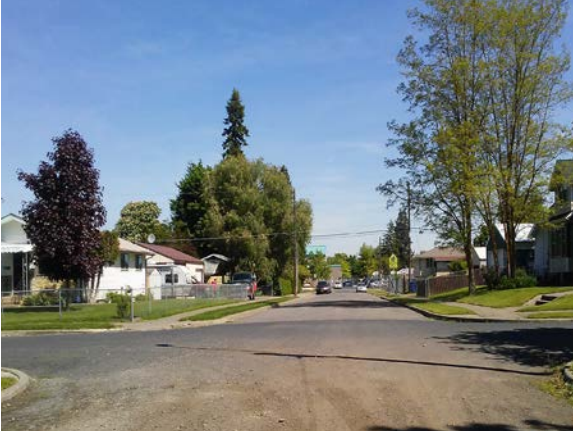
Unpaved section of North Pittsburg Street.
