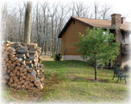
Neatly Stacked Wood Away From House Is Not A Violation!
