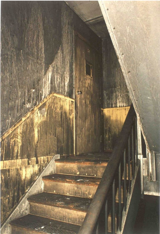
Three people died in this stairwell because of a broken bolt on a fire door.
