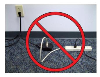
Too many people think of extension cords as permanent fixtures. In fact, OSHA regulations only allow extension cords as **temporary** wiring for up to 90 days! Extension cords used to energize power strips create an additional fire hazard because electrical resistance increases with increased power cord length. The increased resistance also increases heat generation with the accompanying risk of equipment failure and fire.
