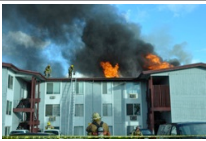
This 3rd Alarm fire on October 31 was caused by an unattended candle. Fifty-four residents were displaced
