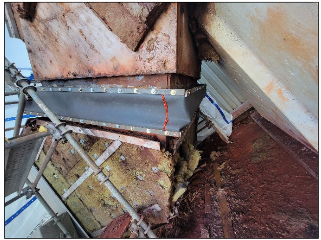
Repairs to ID Fan Outlet Duct
