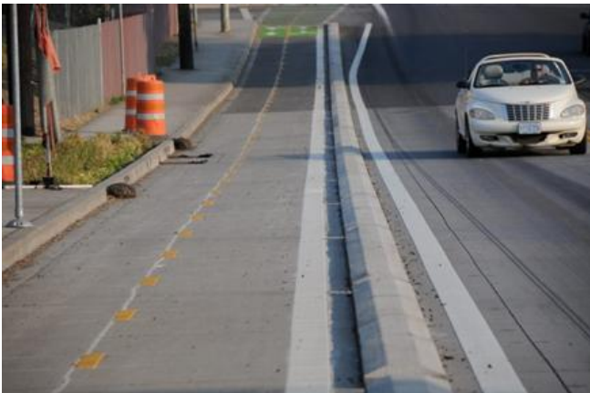
Narrow or Wide Concrete Curbs Image source: Portland's latest protected bikeway goes through an industrial zone on city's northern edge – BikePortland
