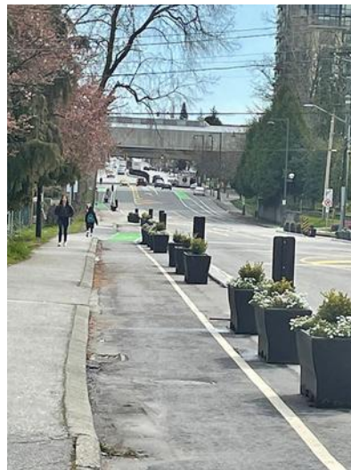
Planters Source: Bike Lanes & Crosswalk Applications | Sybertech Waste
