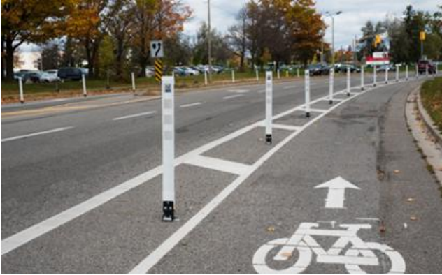
Frequent Flex Posts – City of Toronto, ON Source: Layout - Bicycle lane - bike lane - cycle track - multi-use path flexible bollard - delineator – post
