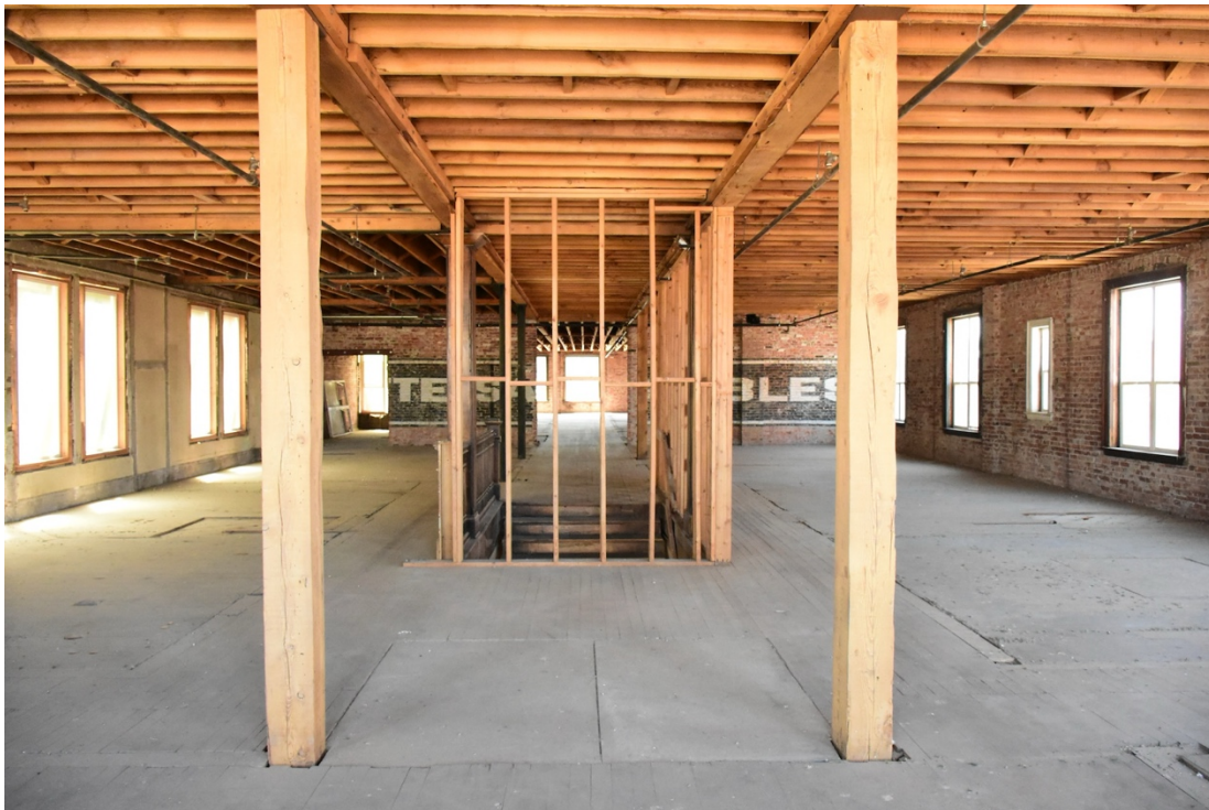
14. Jefferson 3rd floor north section, looking south from north wall
