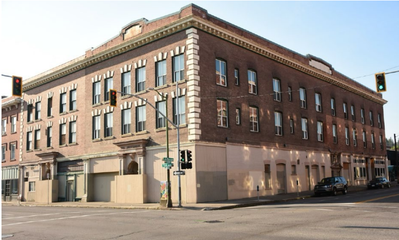
Figure 1: Norman-Jefferson - Northwest corner, looking southeast
