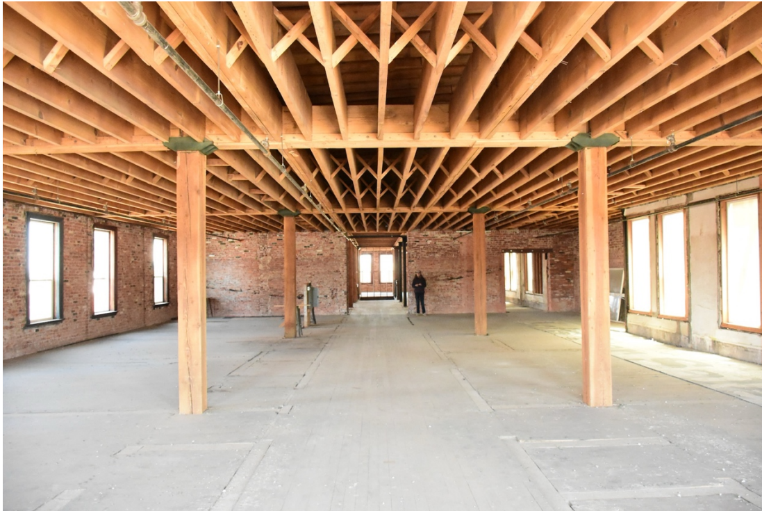
15. Jefferson 3rd floor south section, looking north from south wall
