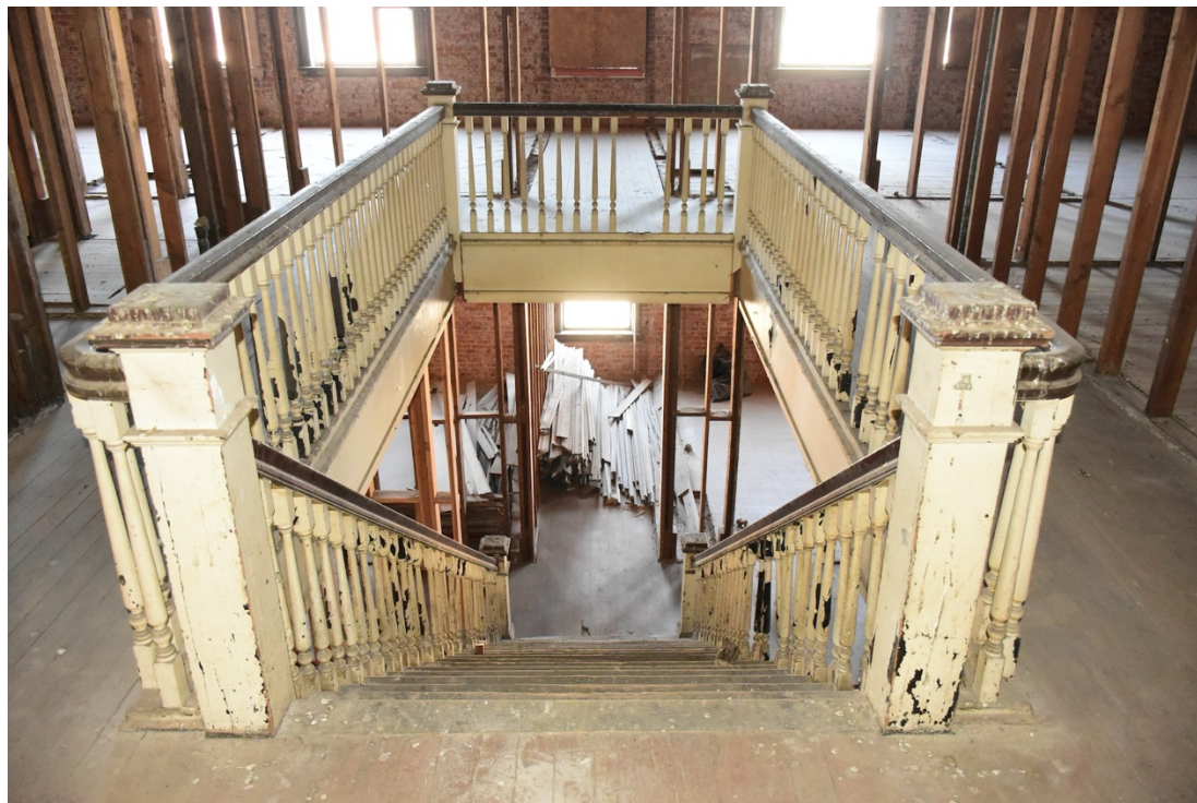
18. Norman 3rd floor, looking north at central stairwell
