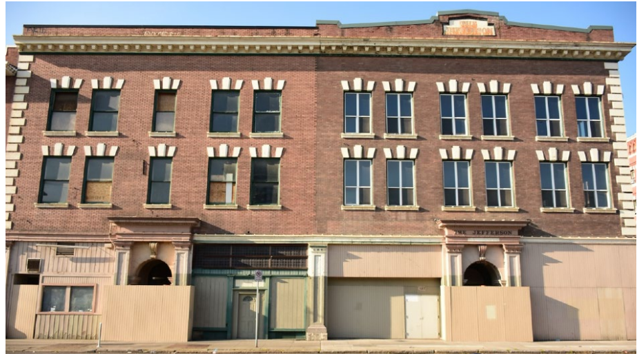
Figure 2: Norman-Jefferson - Front facade, looking south
