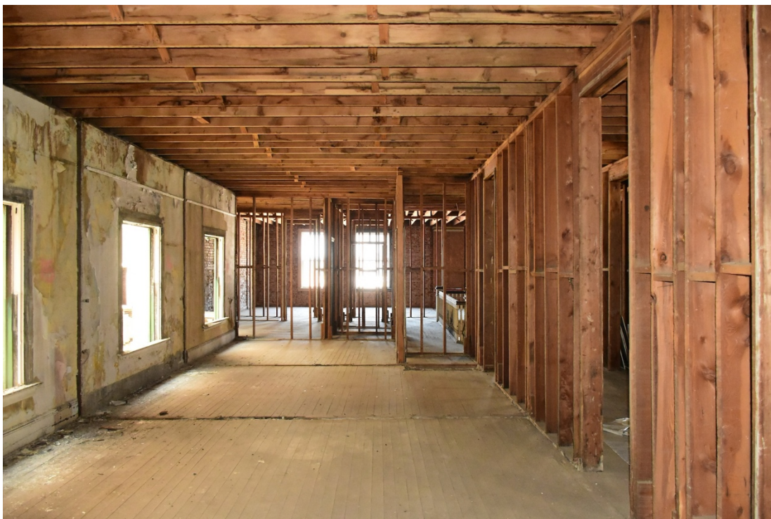
16. Norman 3rd floor, west side, looking north at lightwell and original hallway framing
