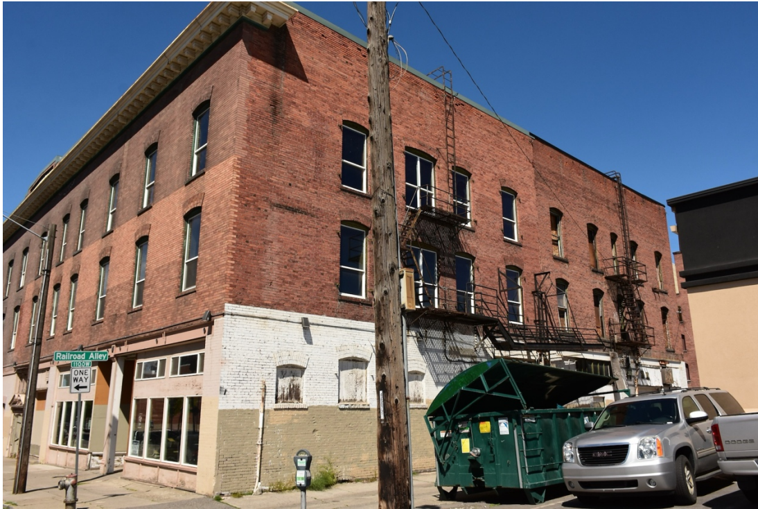
7. Jefferson-Norman - Rear (south) facade, looking northeast
