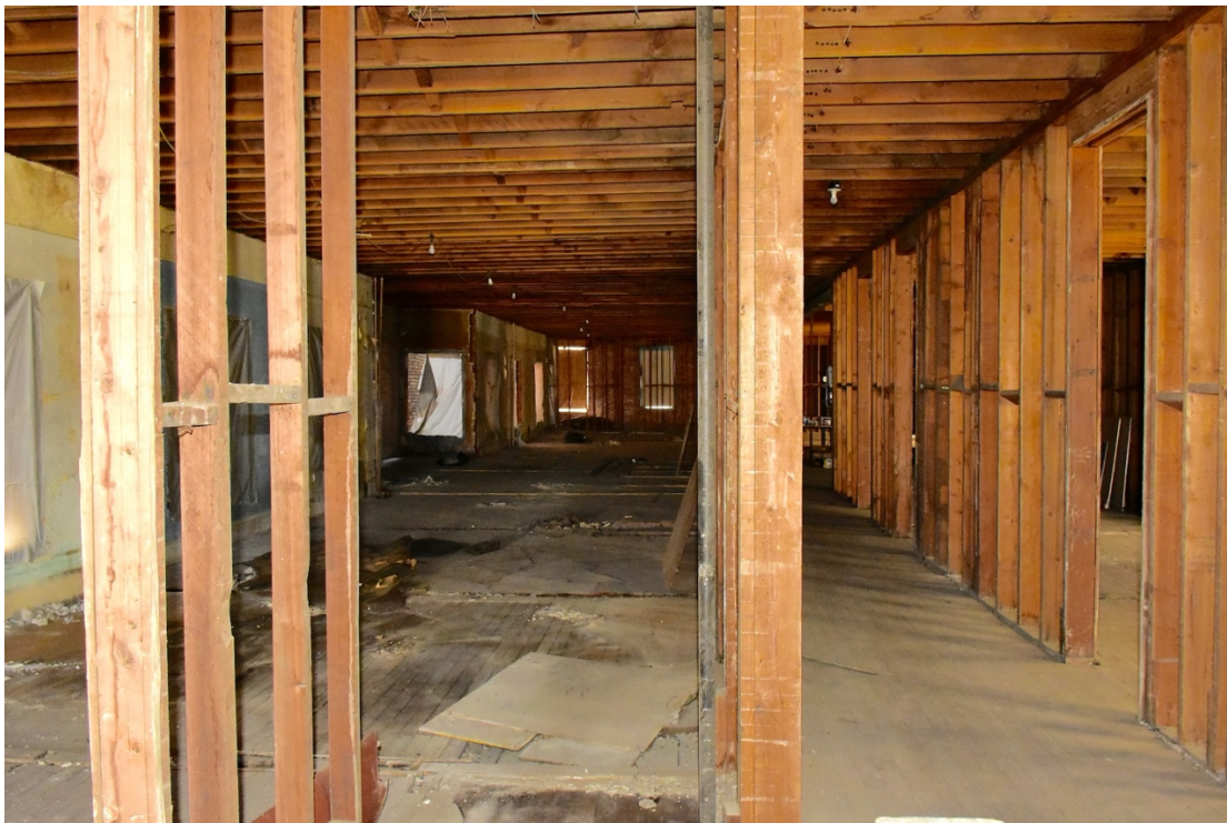
20. Norman 2nd floor, looking south along central hallway
