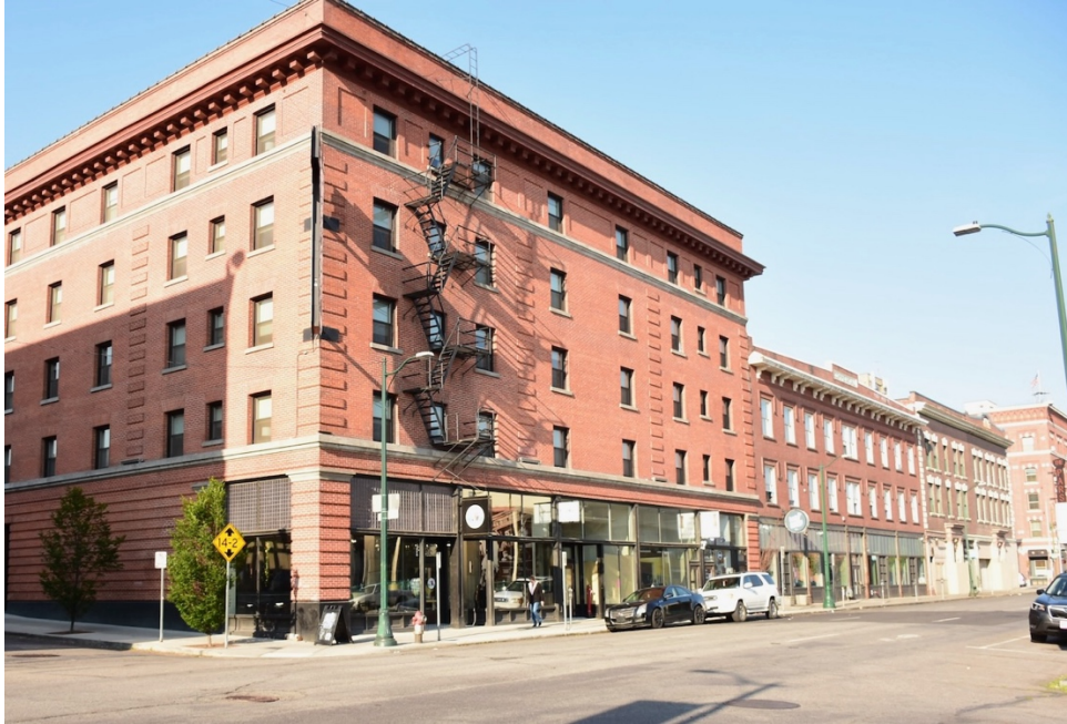
5. Norman-Jefferson - Context along First Avenue, looking southwest
