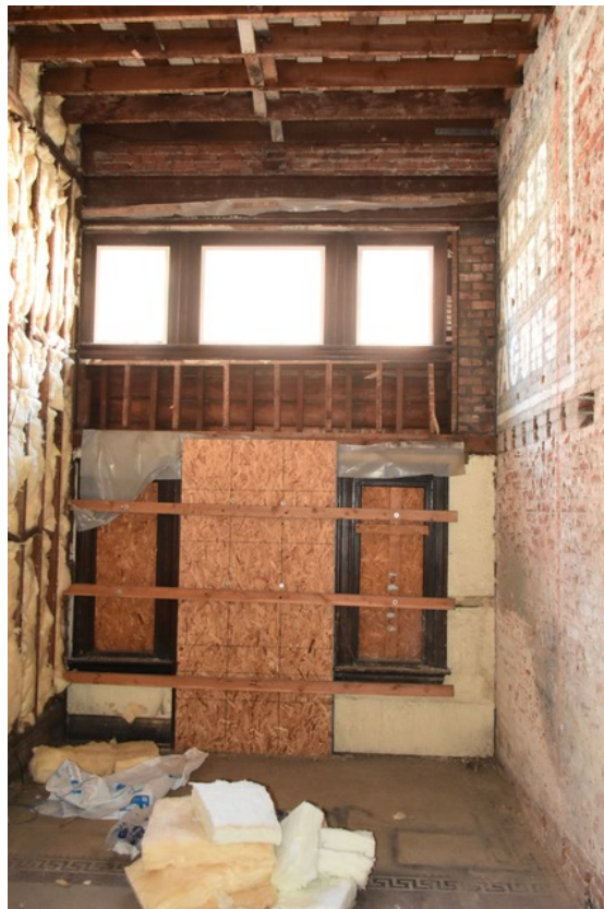
26. Jefferson First Floor - Original entry to south section on west wall, looking west
