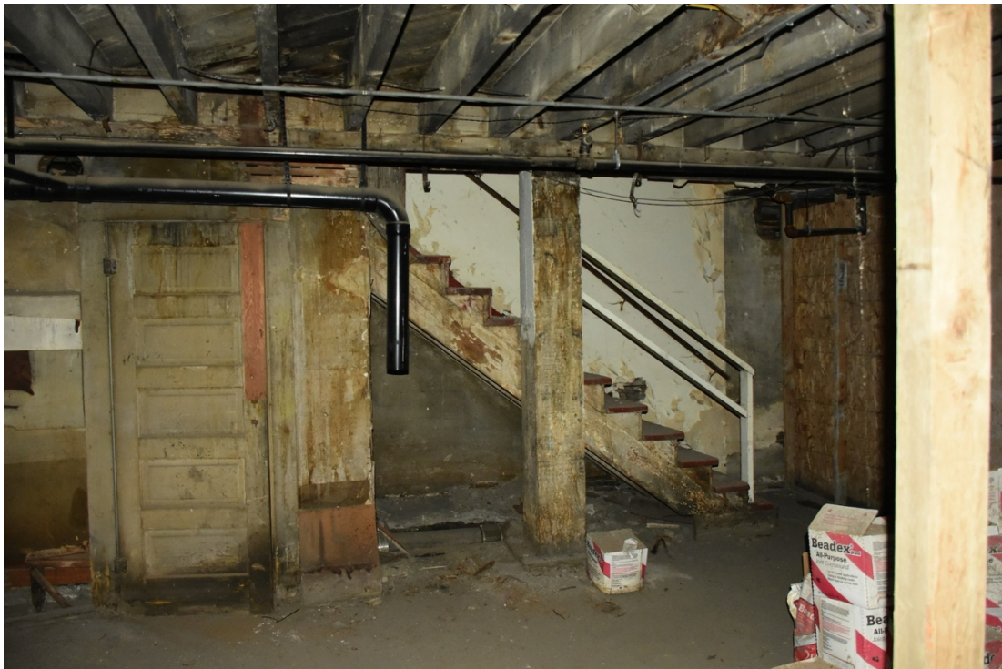
6. Jefferson - Basement on east side with stairs to first floor, looking west
