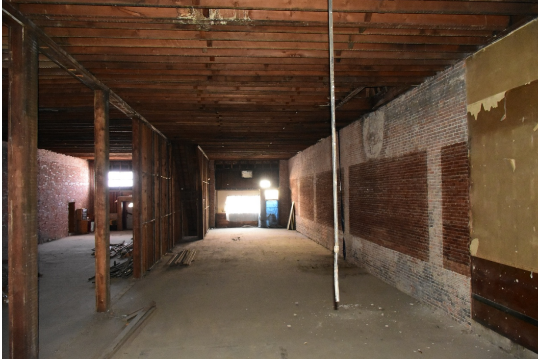
23. Norman 1st floor - looking north along east bay and east wall
