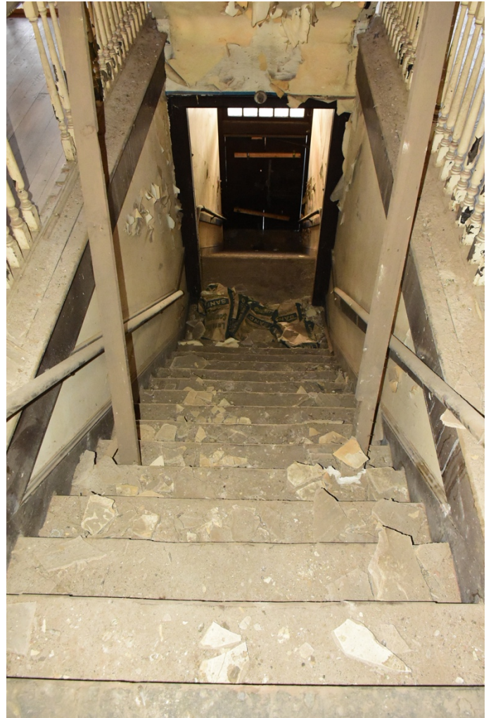
22. Norman 2nd floor central stairwell, looking north down to 1st floor
