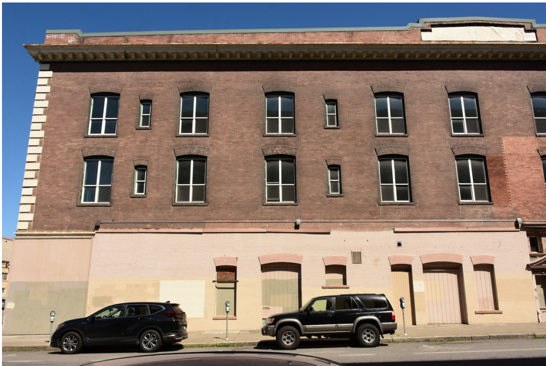
12. Jefferson - west facade, north section, looking east
