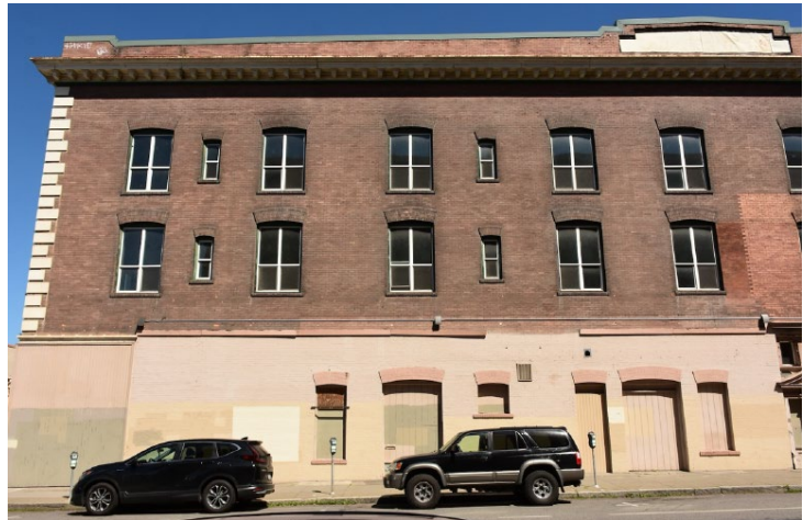
Figure 6: Jefferson - west facade, north section
