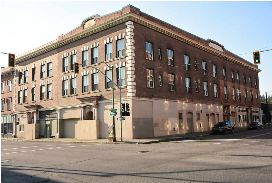
2. Norman-Jefferson - Northwest corner, looking southeast
