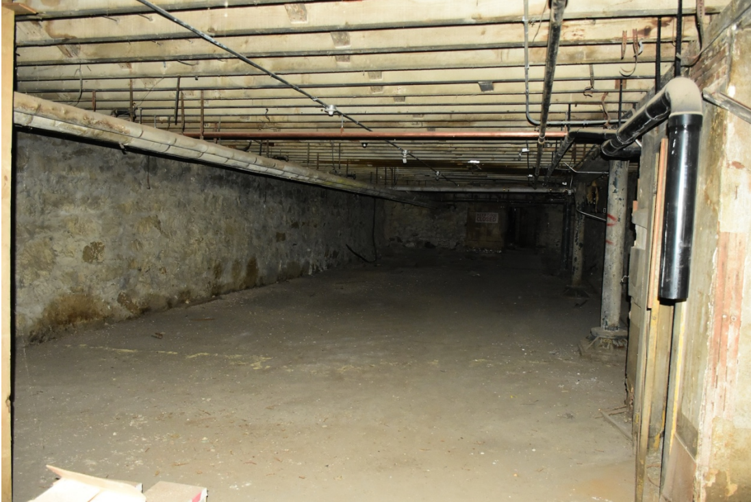
7. Jefferson – Typical basement on east side, looking south
