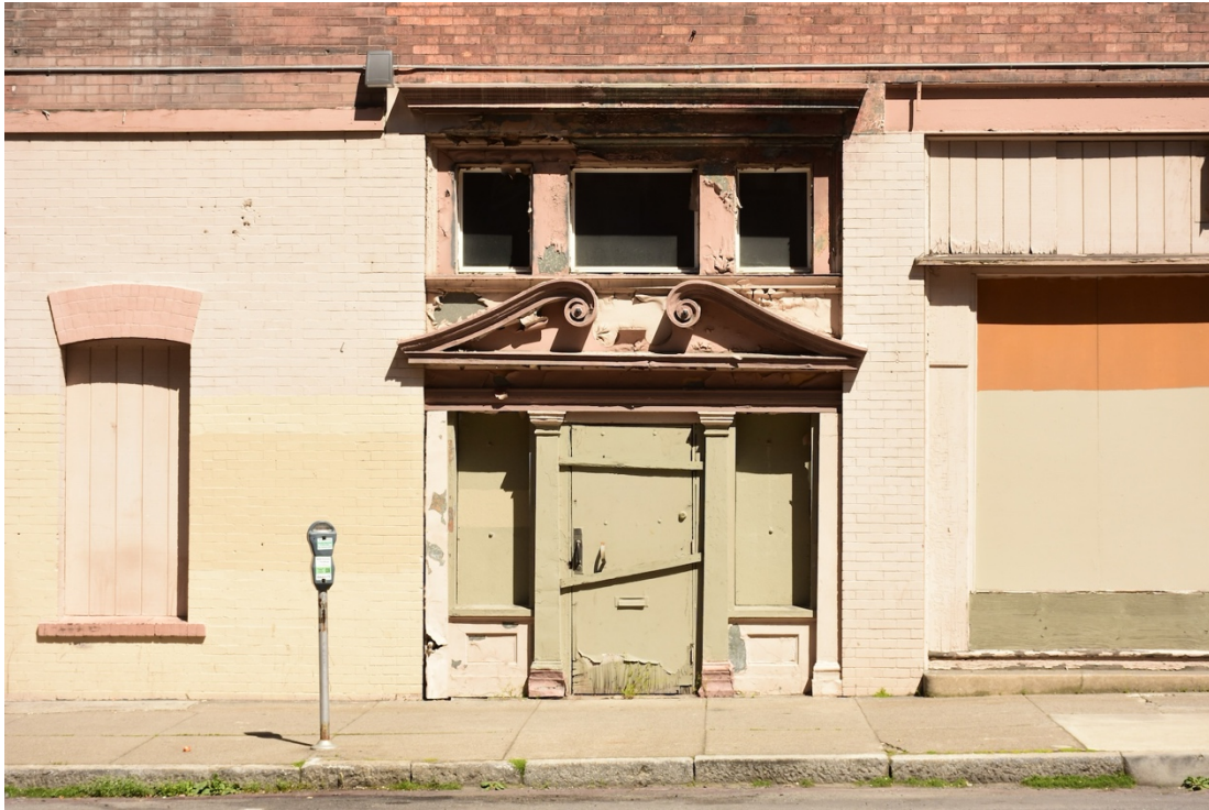
13. Jefferson - West facade, main entrance, looking east
