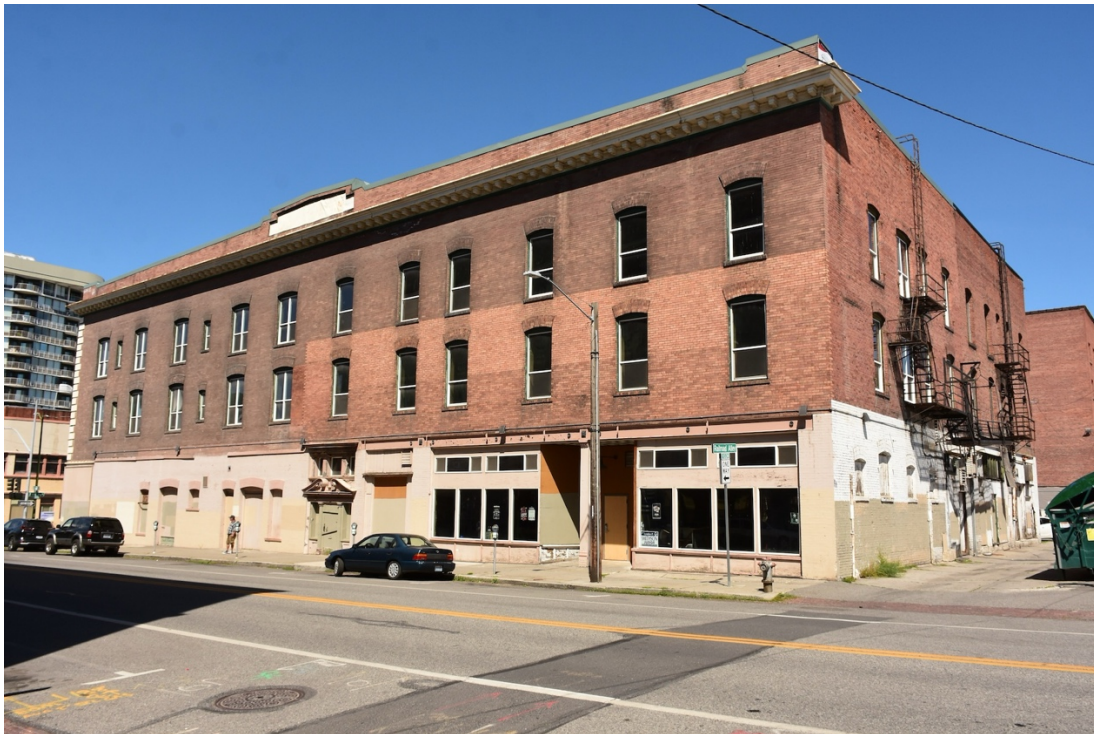
6. Jefferson - Southwest corner and west facade, looking northeast
