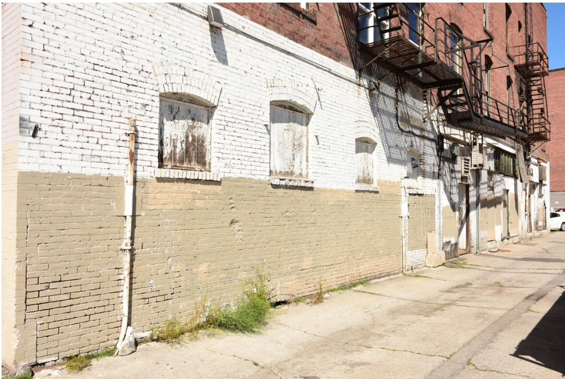
18. Jefferson - southwest corner looking northeast along rear facade of Jefferson and Norman
