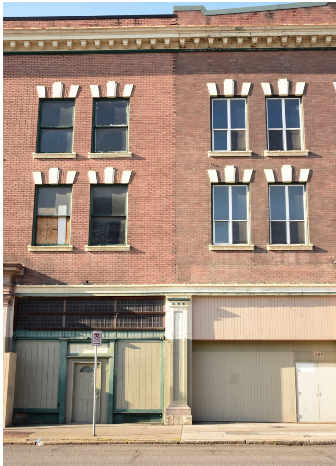
10. Norman-Jefferson - Detail at juncture of buildings
