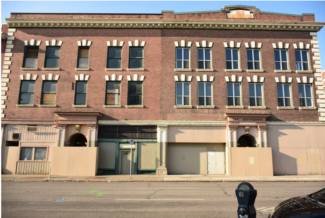
3. Norman-Jefferson - Front facade, looking south
