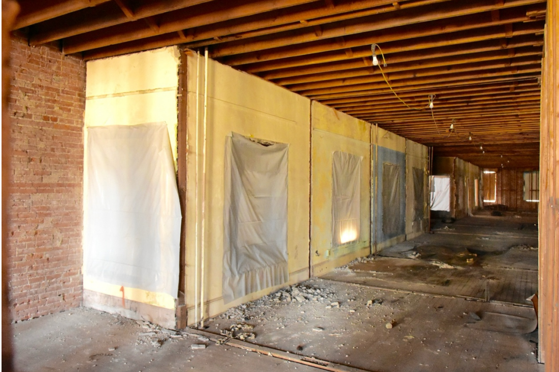
19. Norman 2nd Floor - east wall northerly and southerly light wells, looking south
