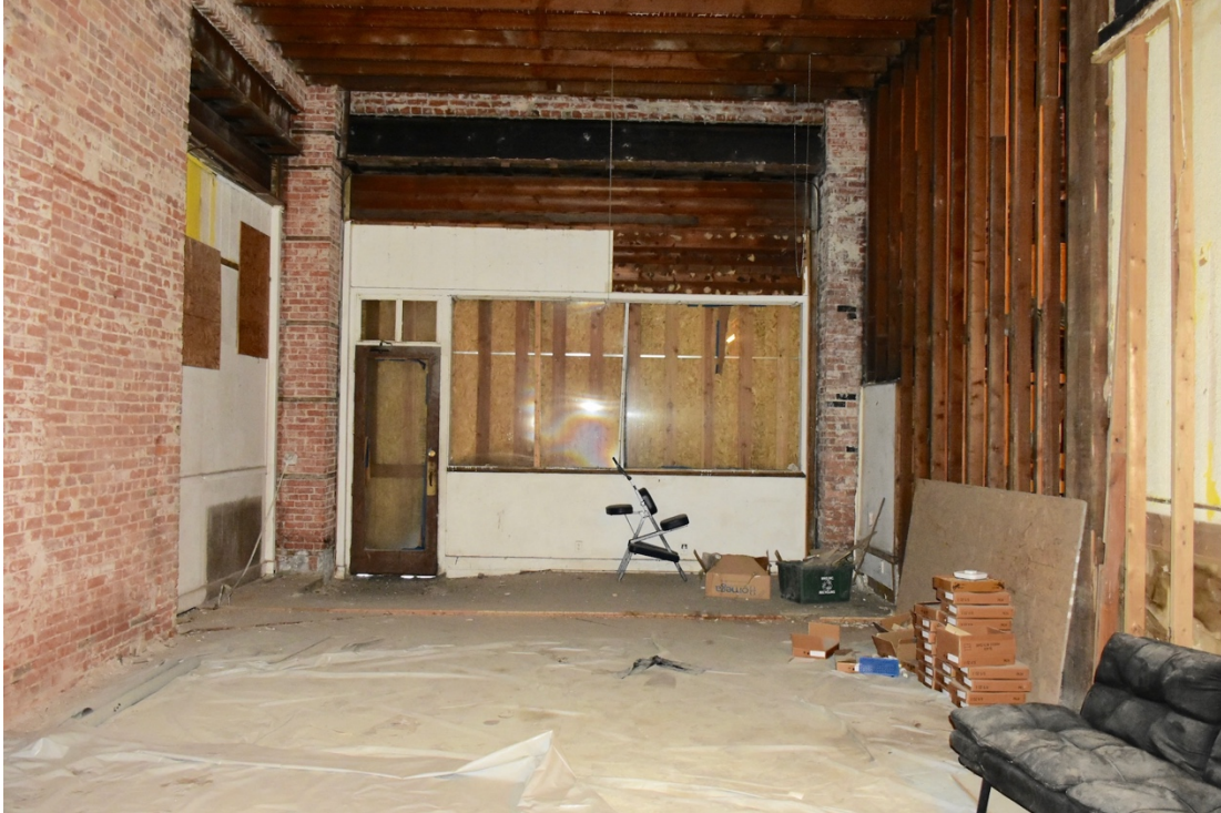
5. Jefferson First Floor - north section, looking north along west wall toward front
