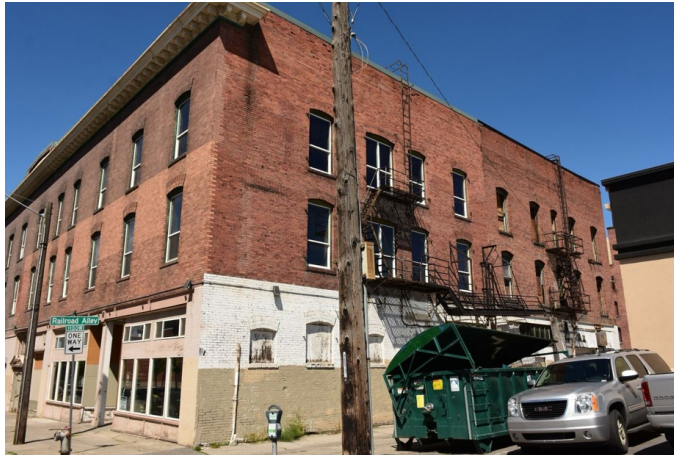
Figure 7: Jefferson-Norman - Rear (south) facade, looking northeast
