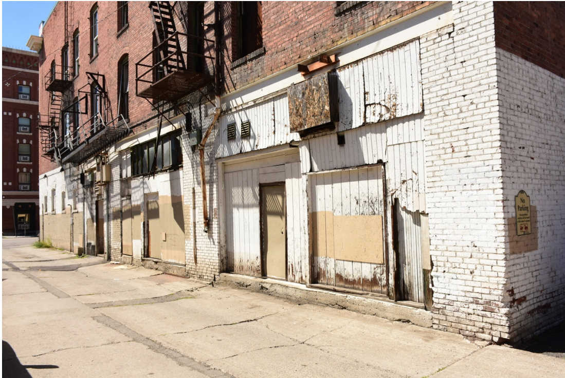
17. Norman - southeast corner, looking northwest along rear facade of Norman and Jefferson
