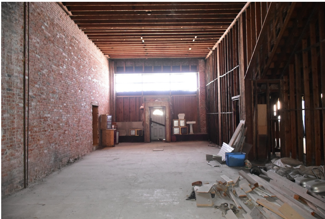
24. Norman 1st floor, looking north along west wall
