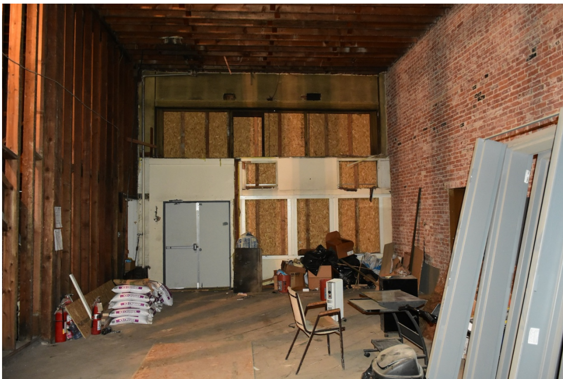
4. Jefferson - First floor, looking north along east wall
