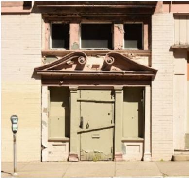
Figure 5: Jefferson - West Facade, main entrance
