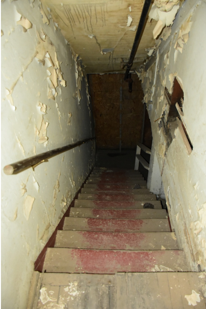
6a. Jefferson - Stairway down to east basement section
