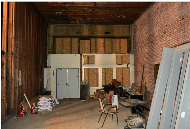
Figure 9: Jefferson - First floor, looking north along east wall
