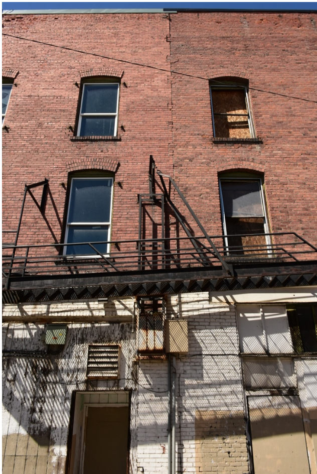
9. Jefferson-Norman - Rear (south) facade at building juncture, looking north
