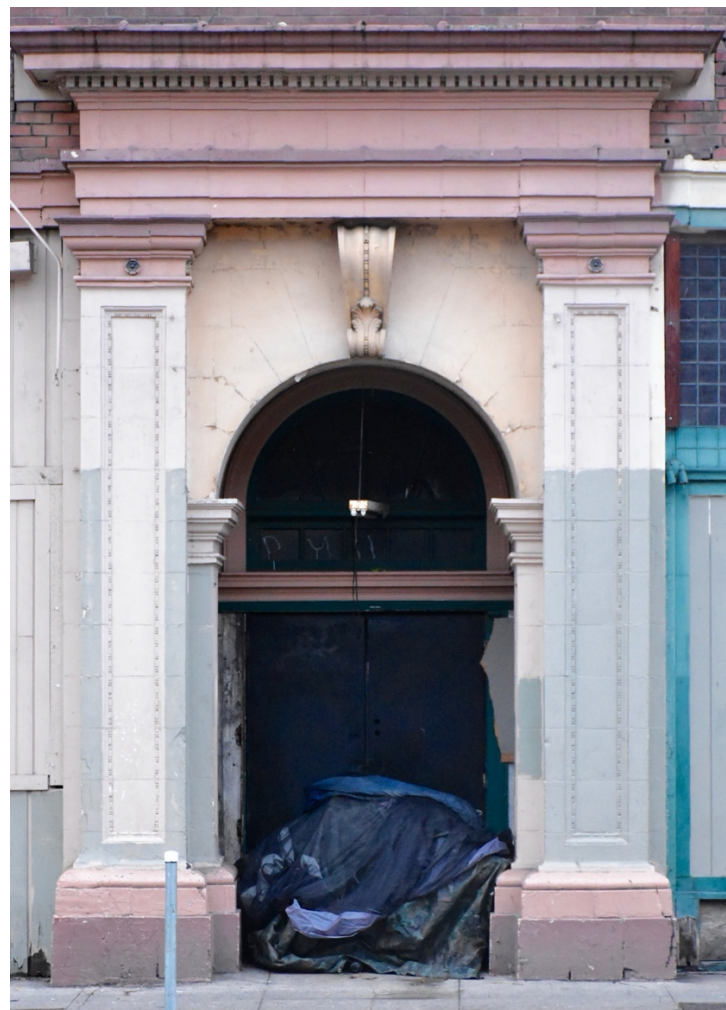
16. The Norman main entrance on 1st Avenue, looking south
