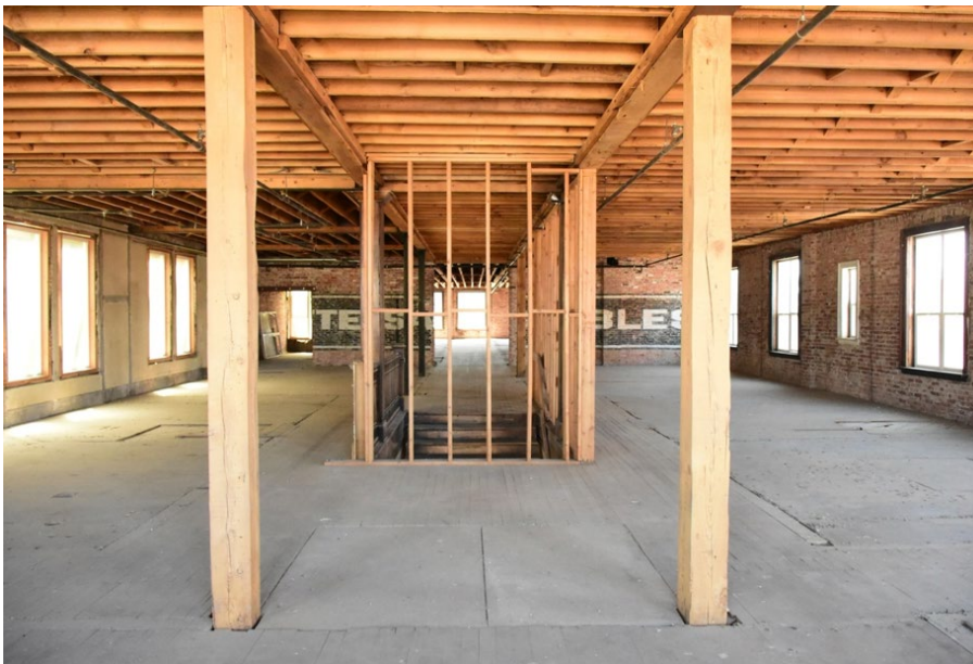
Figure 10: Jefferson 3rd floor north section, looking south from north wall
