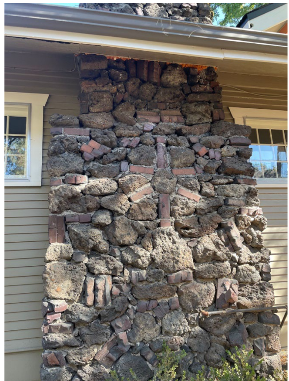
Figure 6: Decorative brick inlay in chimney
