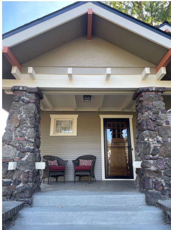
Figure 4: Porch roof and gable in 2024
