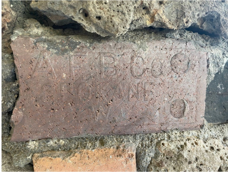
Figure 3: Brick in front porch column stamped with 'AFB Co Spokane WA'
