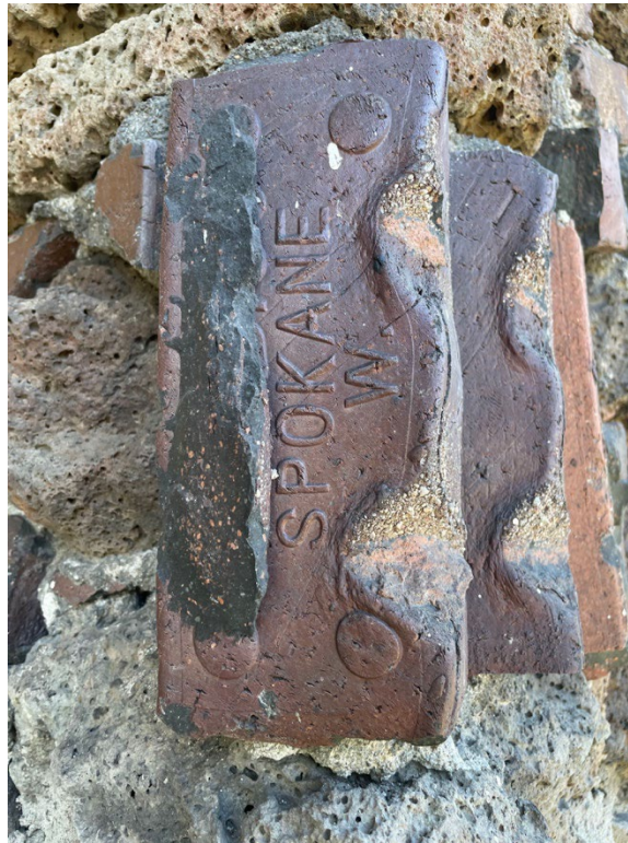
Figure 24: Vertically oriented, misshapen brick in rubblemix column
