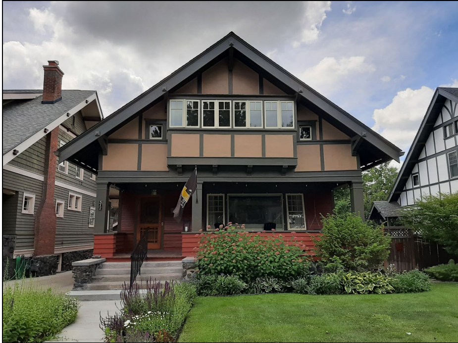
Photo 1 2024 photograph of the north façade of the Mulligan-Brazeau House
