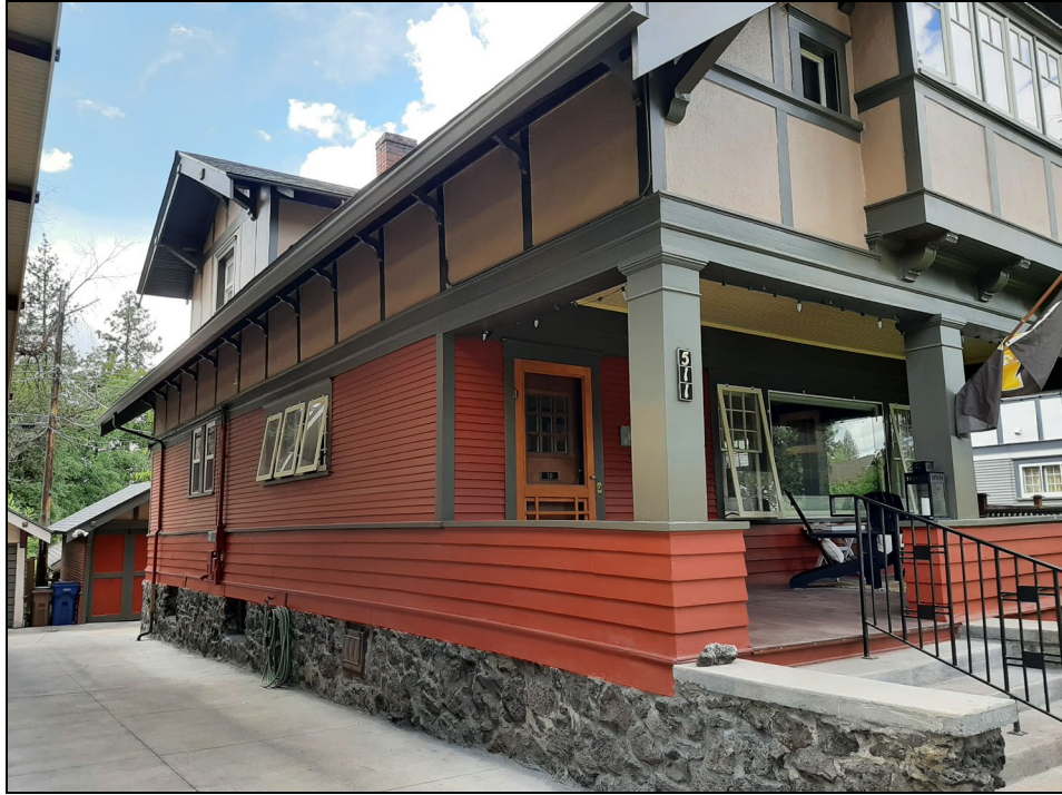
Photo 3 2024 photo of east elevation of house and garage behind house
