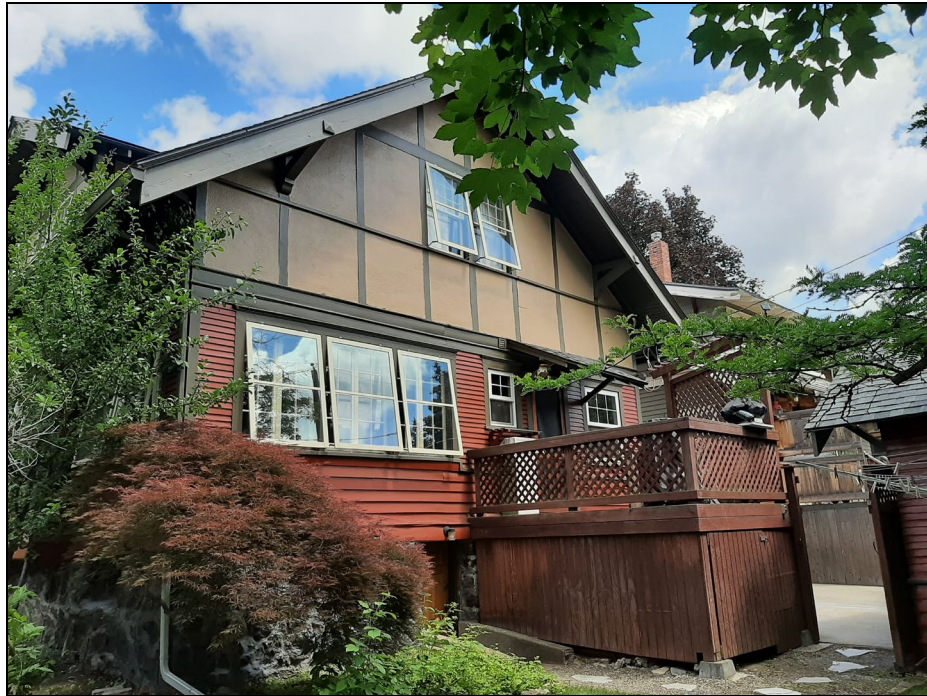
Photo 4 2024 photograph of south rear elevation of house
