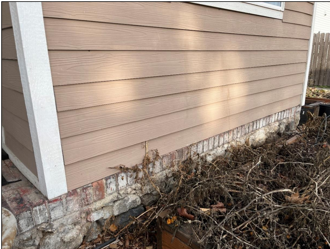
Cook-Abele House rear porch foundation and brick floor where the porch is enclosed on the east end, 12/15/2023. Photo taken by Logan Camporeale SHPO.
