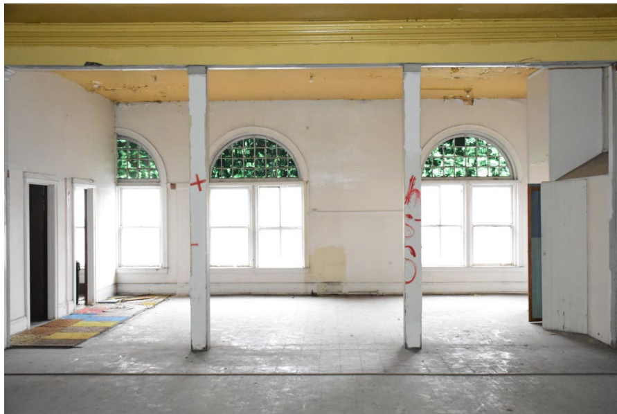
#29. Third floor -north wall, restrooms on west, stair lobby on east
