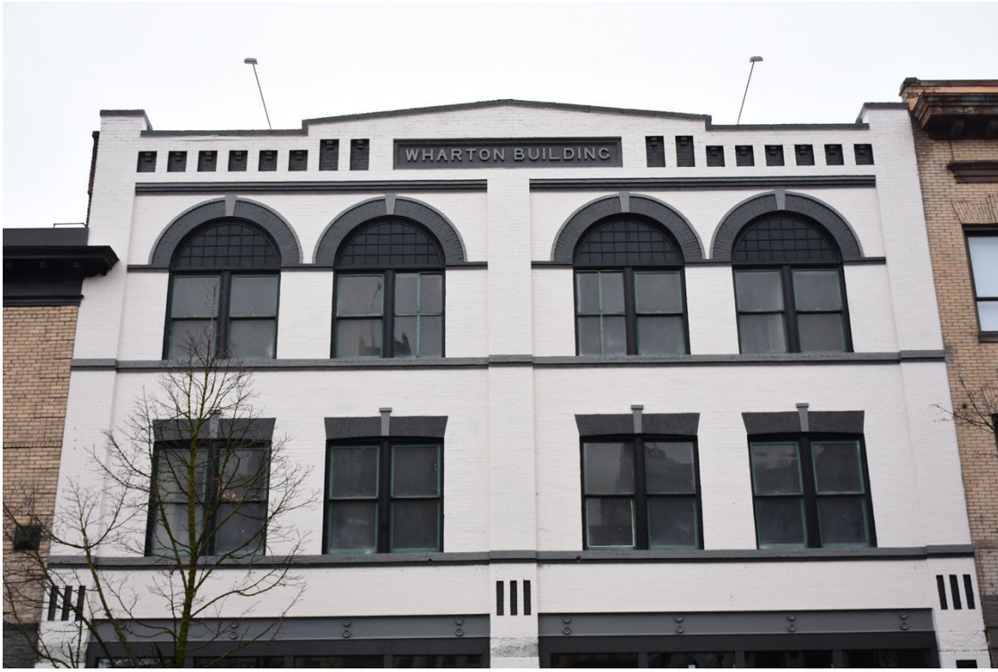
4. Front Facade, looking south
