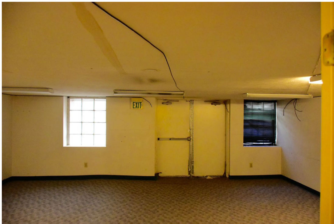
#9. Mezzanine - east side living area/bedroom, looking south
