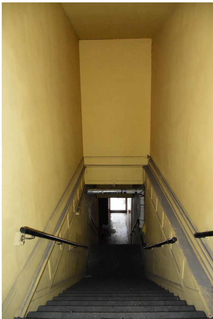
#14. Stairs from second floor to ground floor entry, looking north
