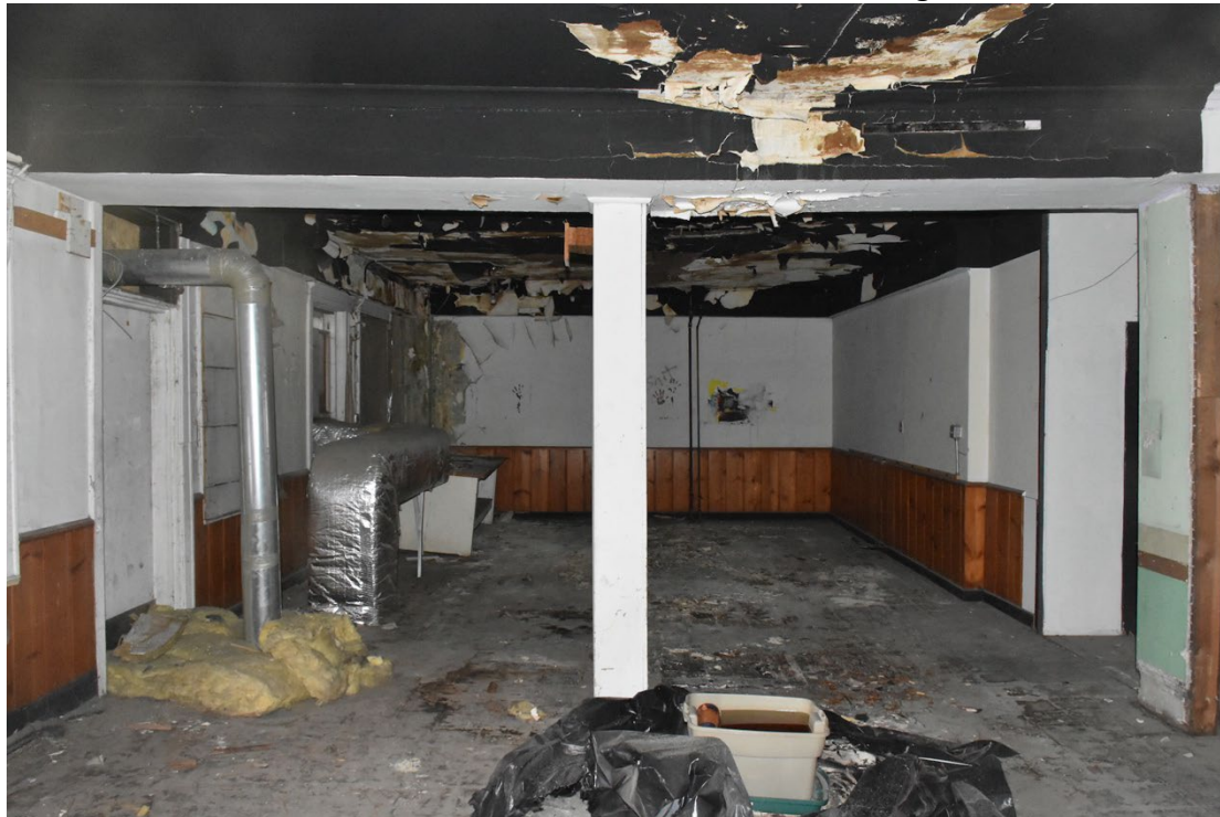
#16. Second floor-southeast corner room, looking south
