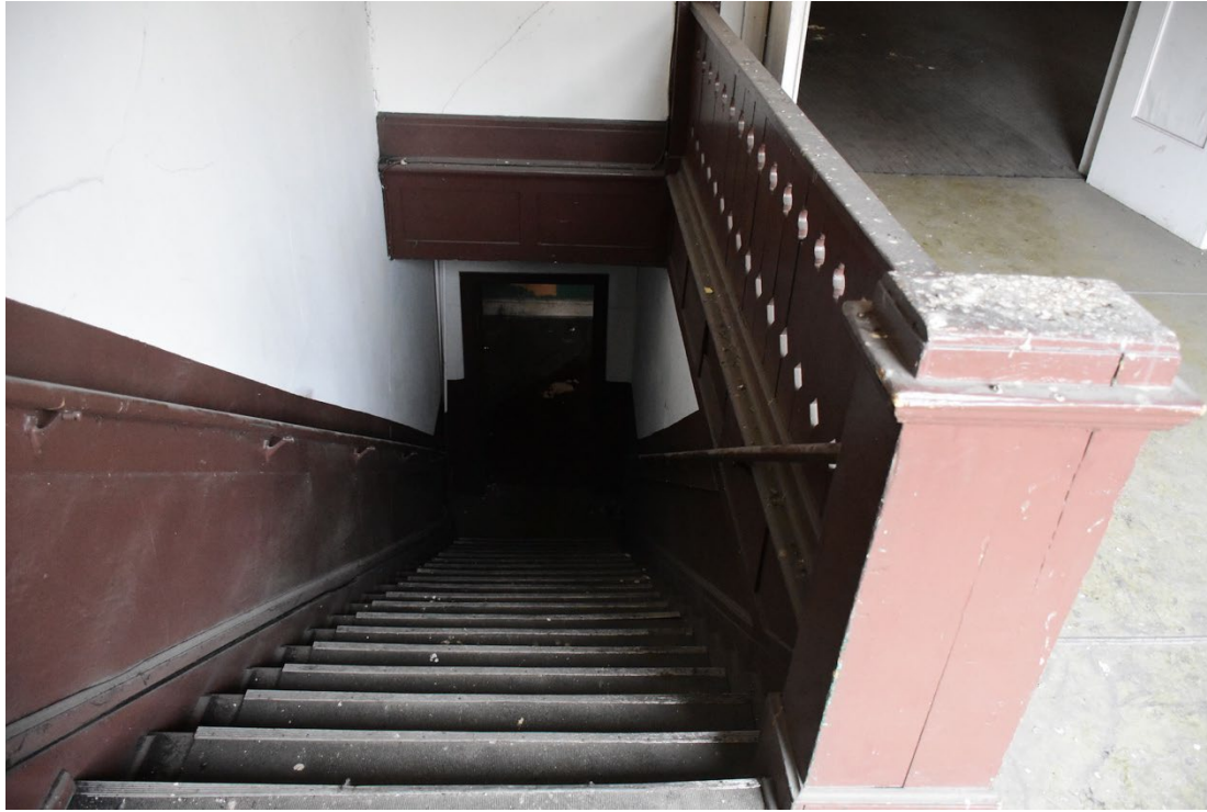
#23. Stairs from second to third floor, looking north
