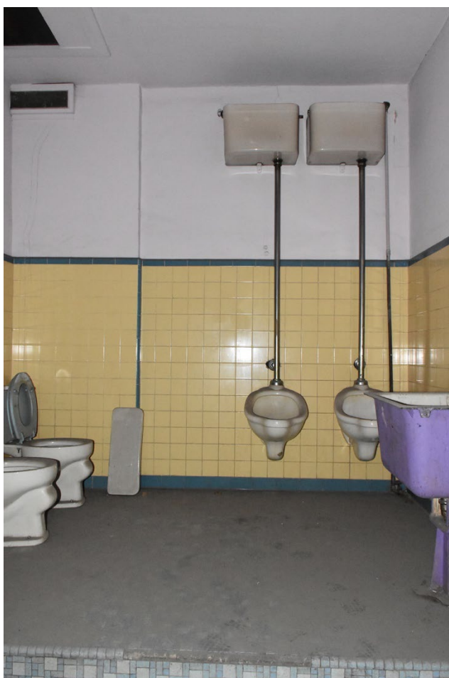
#19. Second floor - typical men's restroom, looking west
