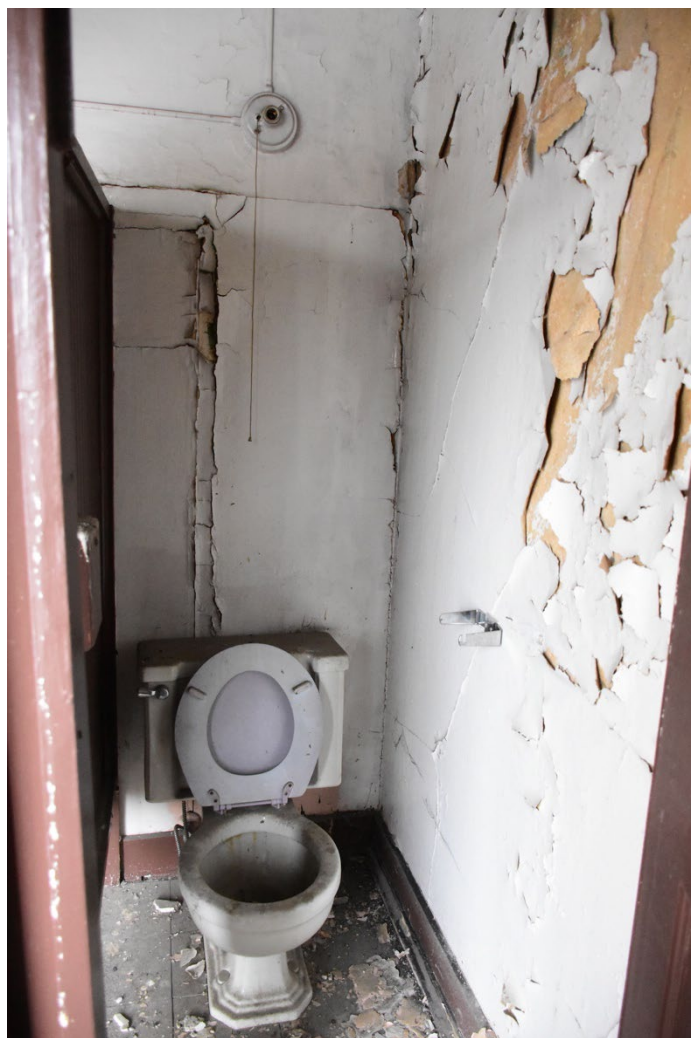
#31. Third floor restroom-toilet, northwest corner
