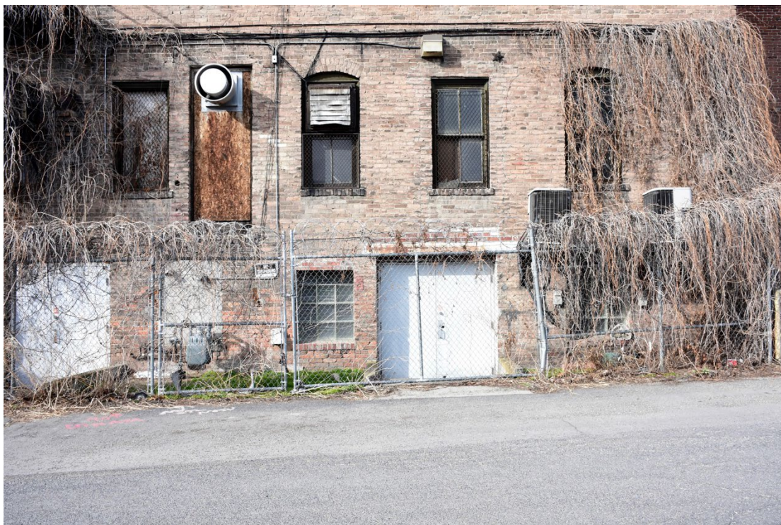
12. Rear facade - detail of windows & doors, looking north
