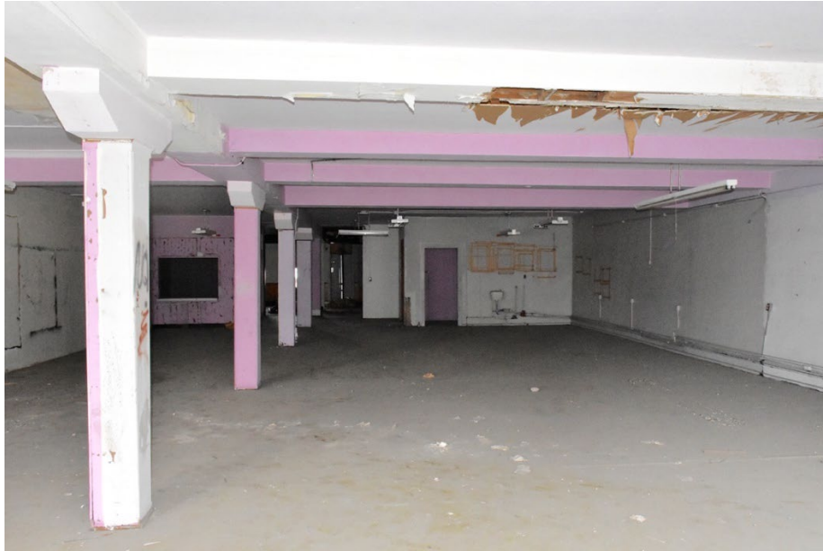
#21. Second floor - lodge hall, looking southeast at east wall
