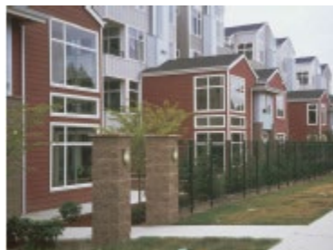
Windows facing street
