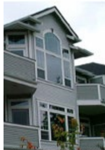
Windows with visually prominent trim
