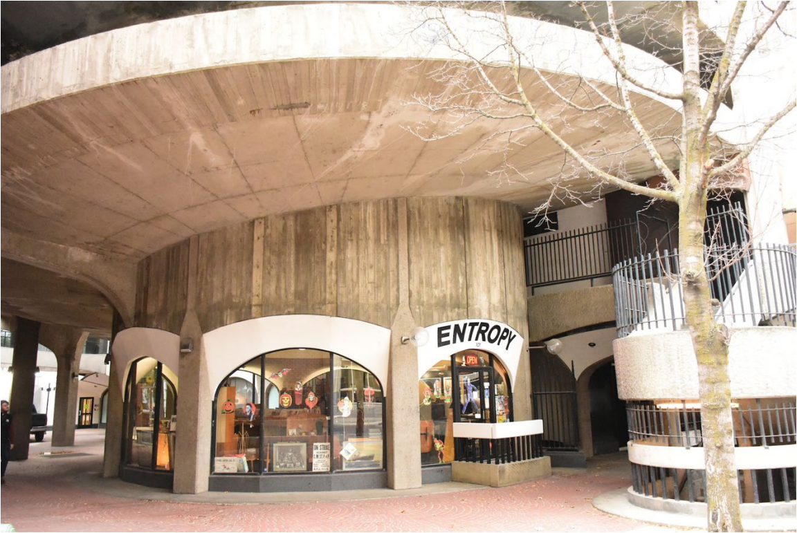
19. Ground floor - southeast corner retail shop beneath spiral ramp, looking northwest (9/2023)
