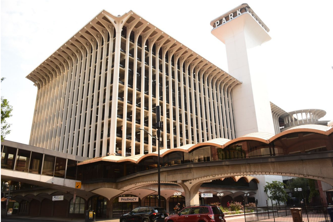
1. Southwest corner, looking northeast at west and south facades (8/2023)
