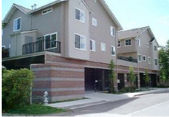
Parking structure at ground level with architectural banding and shrubs
