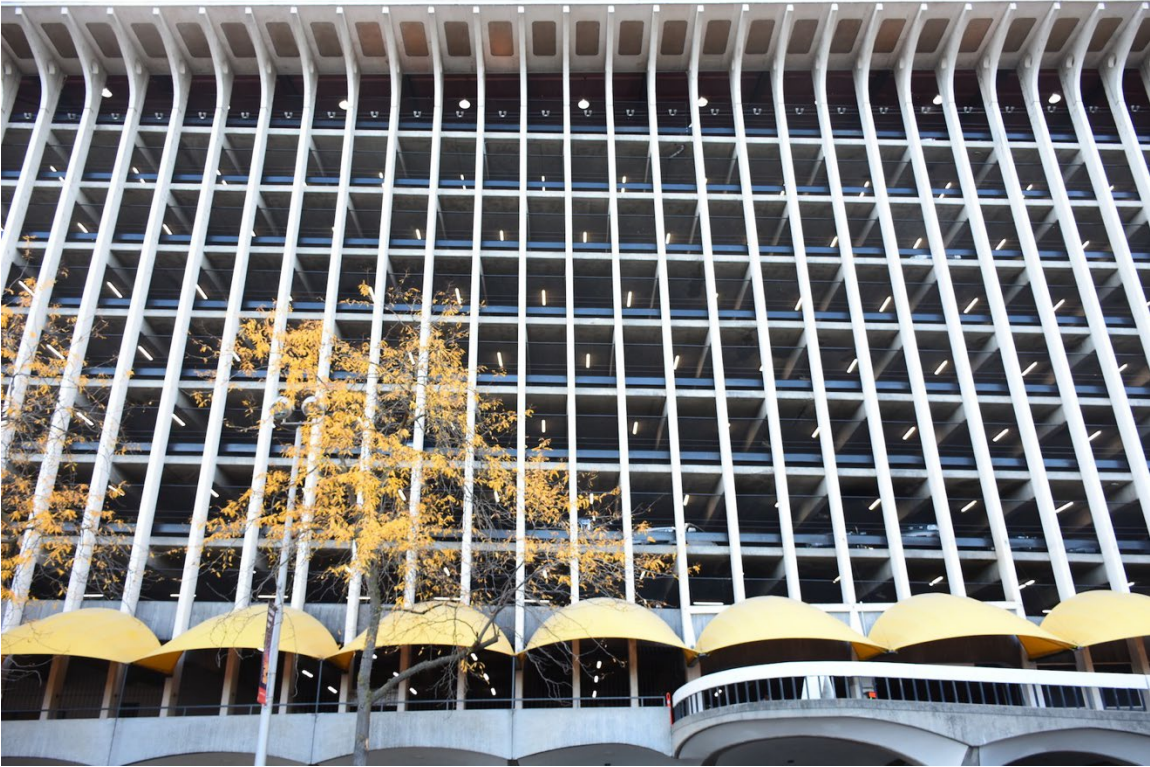
7. North facade, looking south at floors 2 to 10- skywalk to cornice (10/2023)
