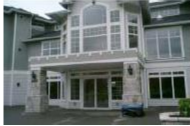
entrance with portico and ornamental treatments
