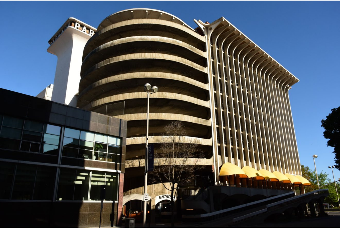
4. Southeast corner, spiral exit ramp, tower, looking northwest (8/2020)
