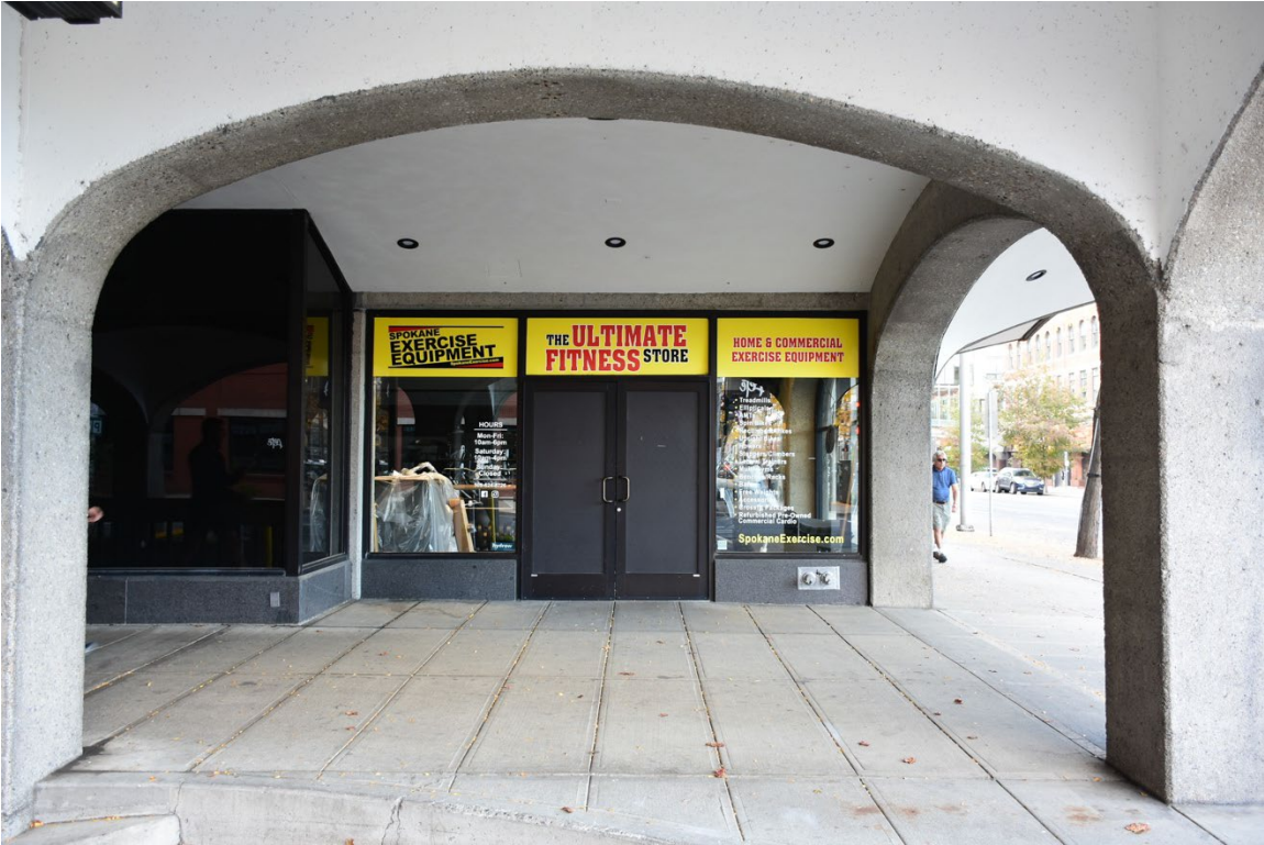
17. East facade- northeast corner entry to retail space, looking west (10/2023)
