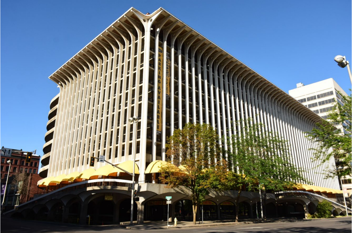
3. Northeast corner, looking southwest at east and north facades (8/2023)
