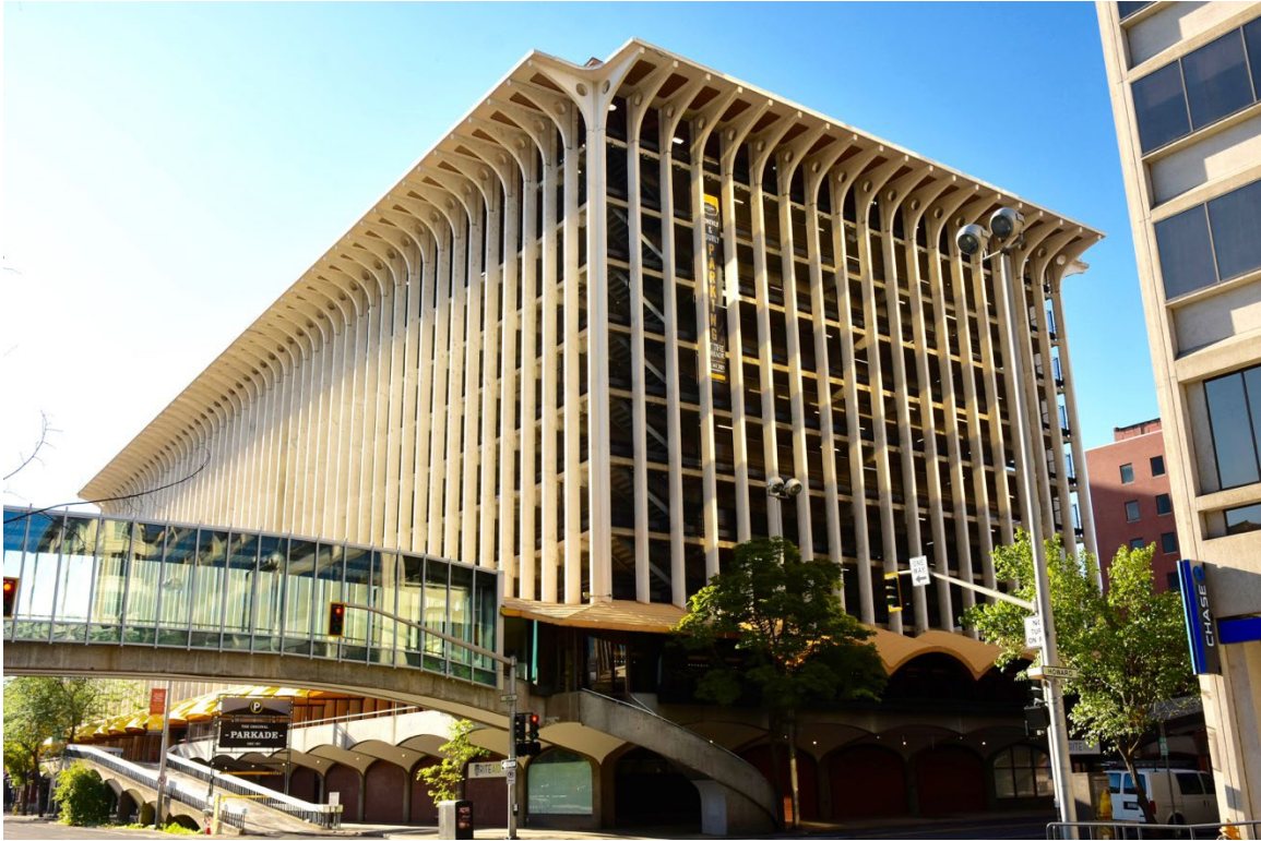
2. Northwest corner, looking southeast at west and north facades (8/2023)
