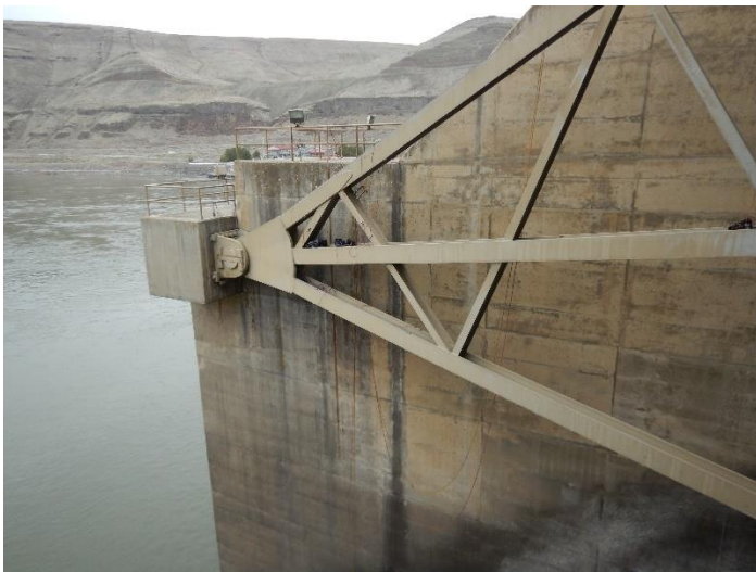
Figure 2 Typical strain transducer installation.
