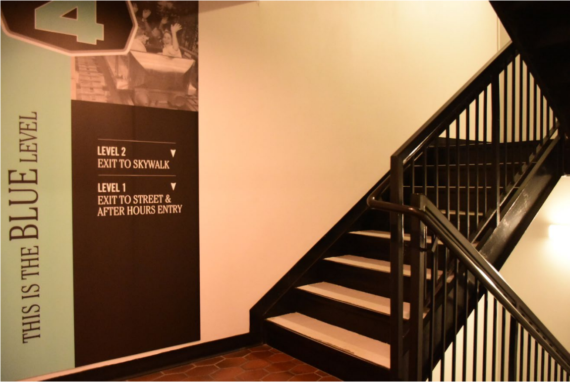
31. Elevator/stair tower – stairs at blue level (level 4) landing looking south (10/2023)
