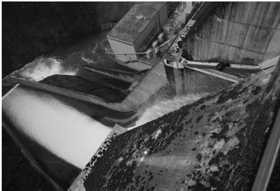
Figure 6 Upper Baker Dam - Puget Sound Energy, Concrete, WA
