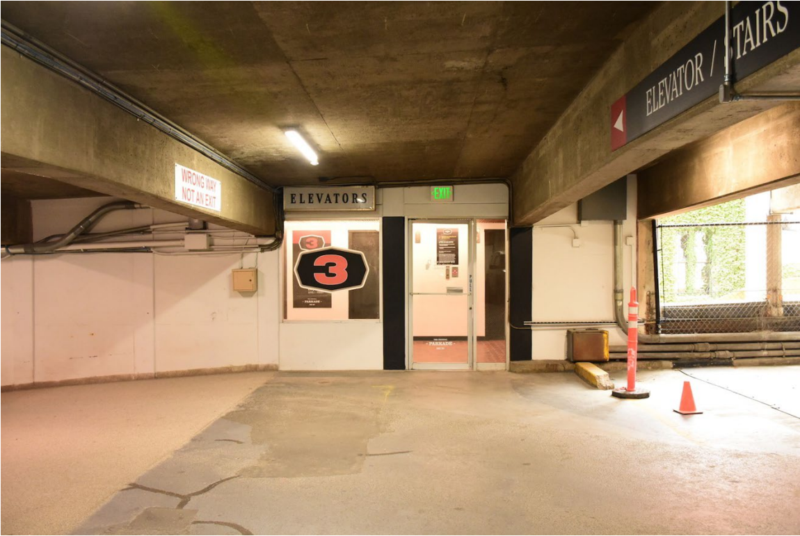
29. Red level (floor 3), looking south across ramp to elevator/stair lobby (10/2023)
