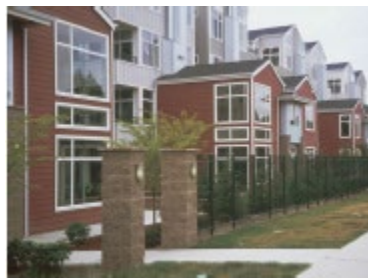
Windows facing street
