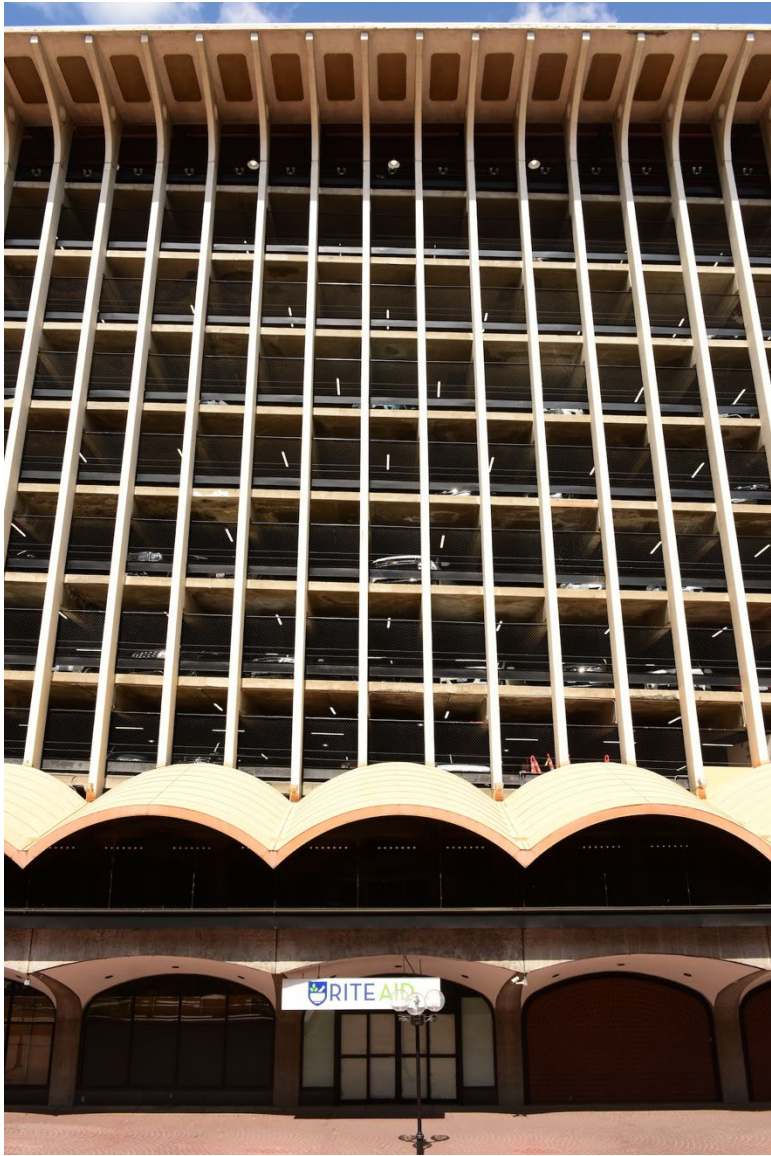
12. South facade west of tower, looking north (9/2023)
