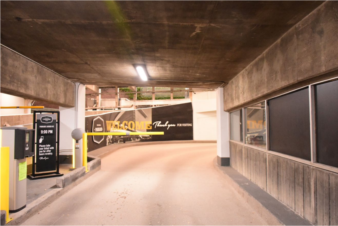
27. Skywalk level entry to parking garage red level, looking south (10/2023)
