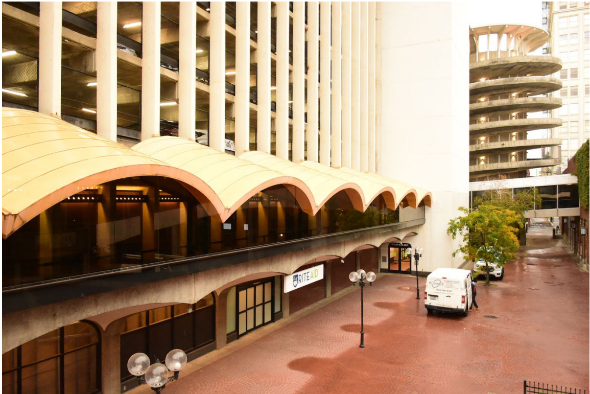
11. South facade skywalk level, looking east at elevator/stair tower and spiral ramp (10/2023)
