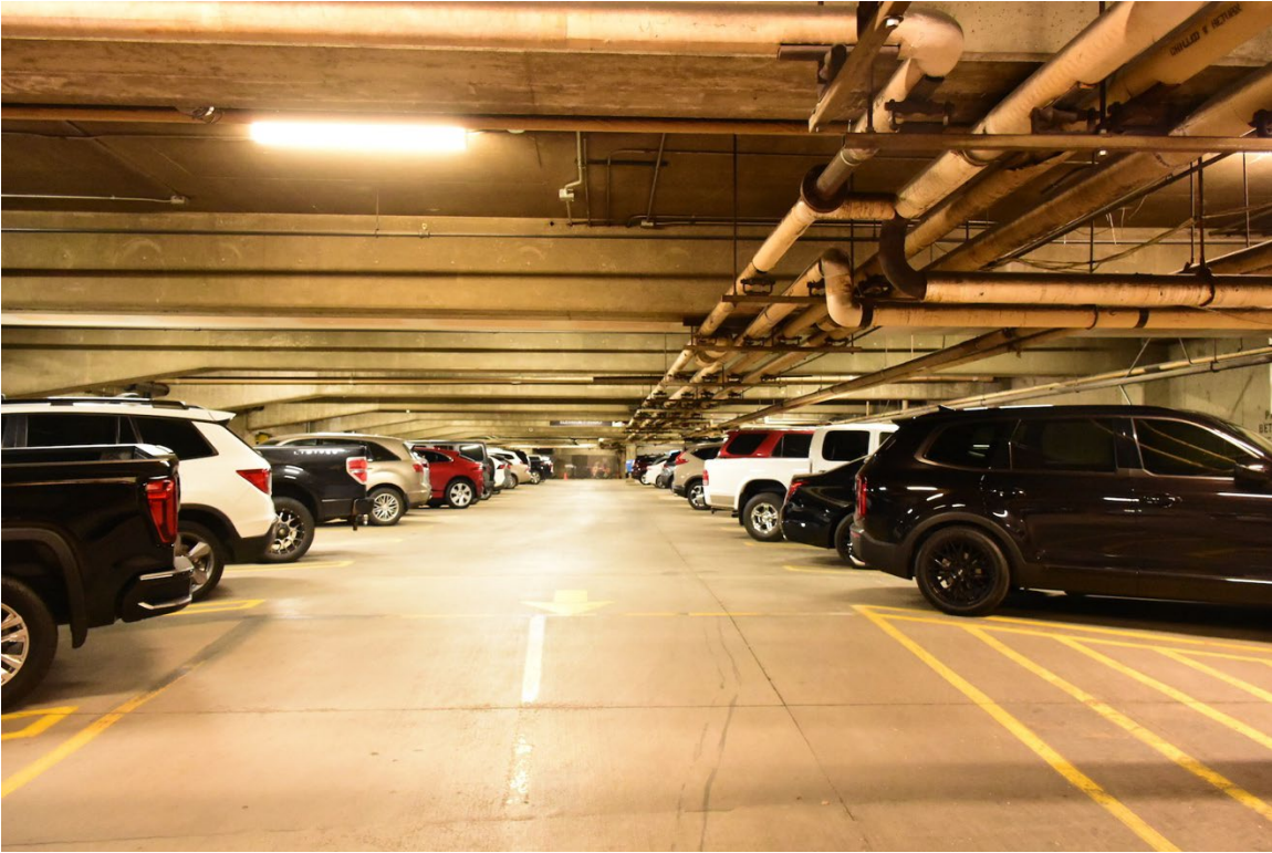
24. Basement parking garage - south lane, looking east (12/2020)
