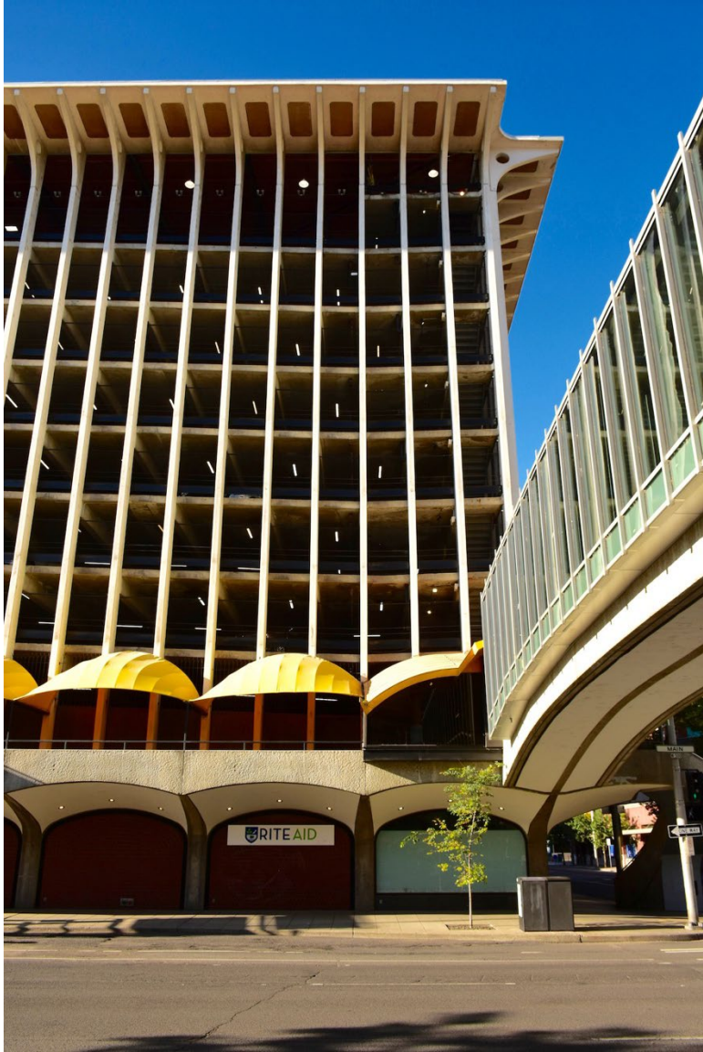
5. West end of north façade, skywalk across Main Avenue on west, looking south (9/2023)
