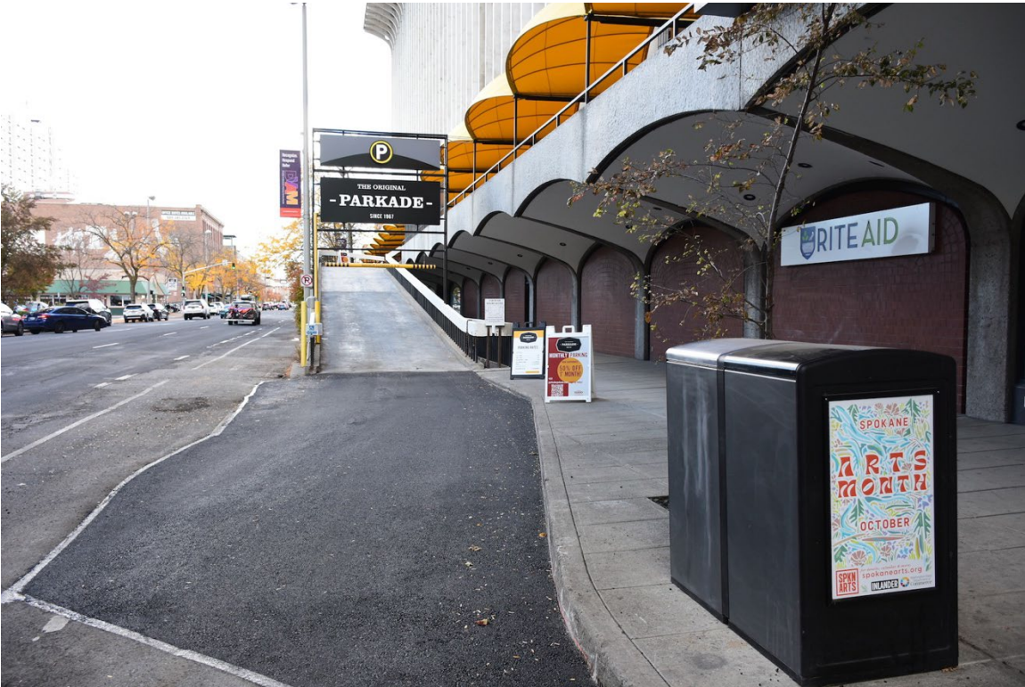
9. North side-Main Avenue entry ramp, looking east (10/2023)
