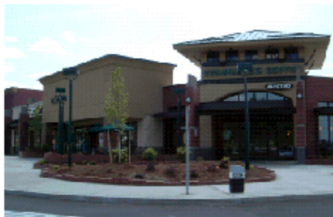
Plaza located at main entrance
