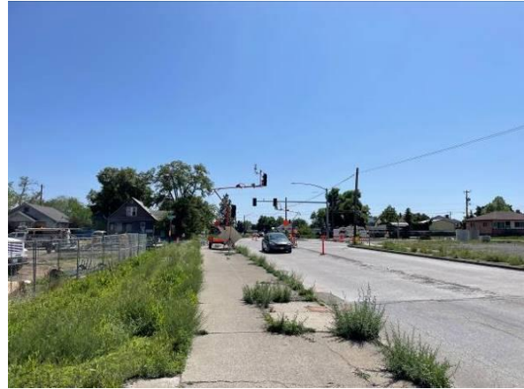
View of North Haven Street Facing South
