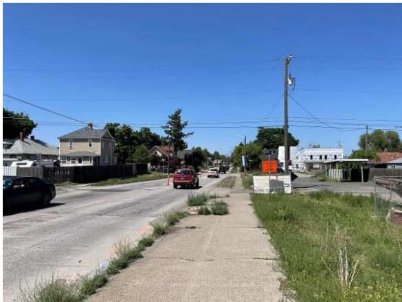
View of North Haven Street Facing North
