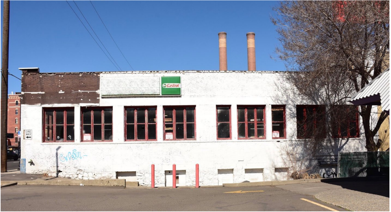
9. South facade - ground floor and basement, looking north
