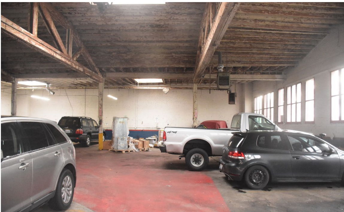
20. Garage, looking east along south wall
