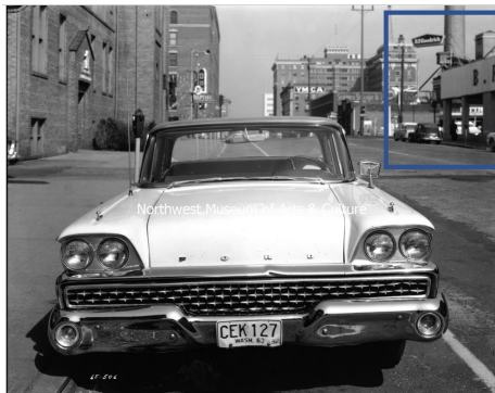
L87-1.506-65 NW MAC JEF Research Archives Libby Collection – 1965 photo showing the porte cochere corner of the Ahrens & Ahrens Building
