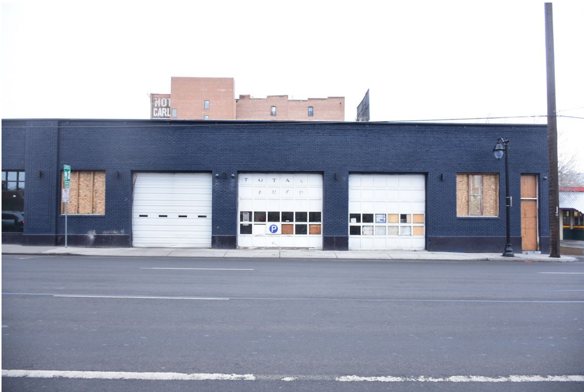
7. West Facade -south half, looking east.
