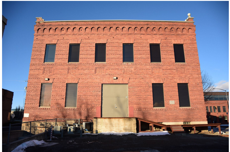
Figure 11: South (rear) elevation
