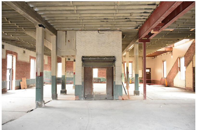
Figure 13: First floor looking north from south wall
