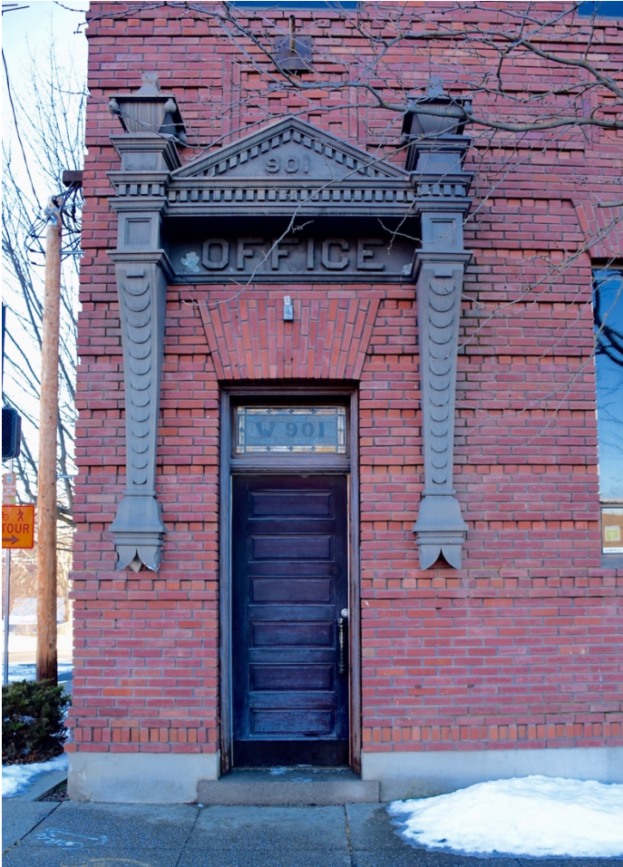
#13. Front Entry, original, looking south
