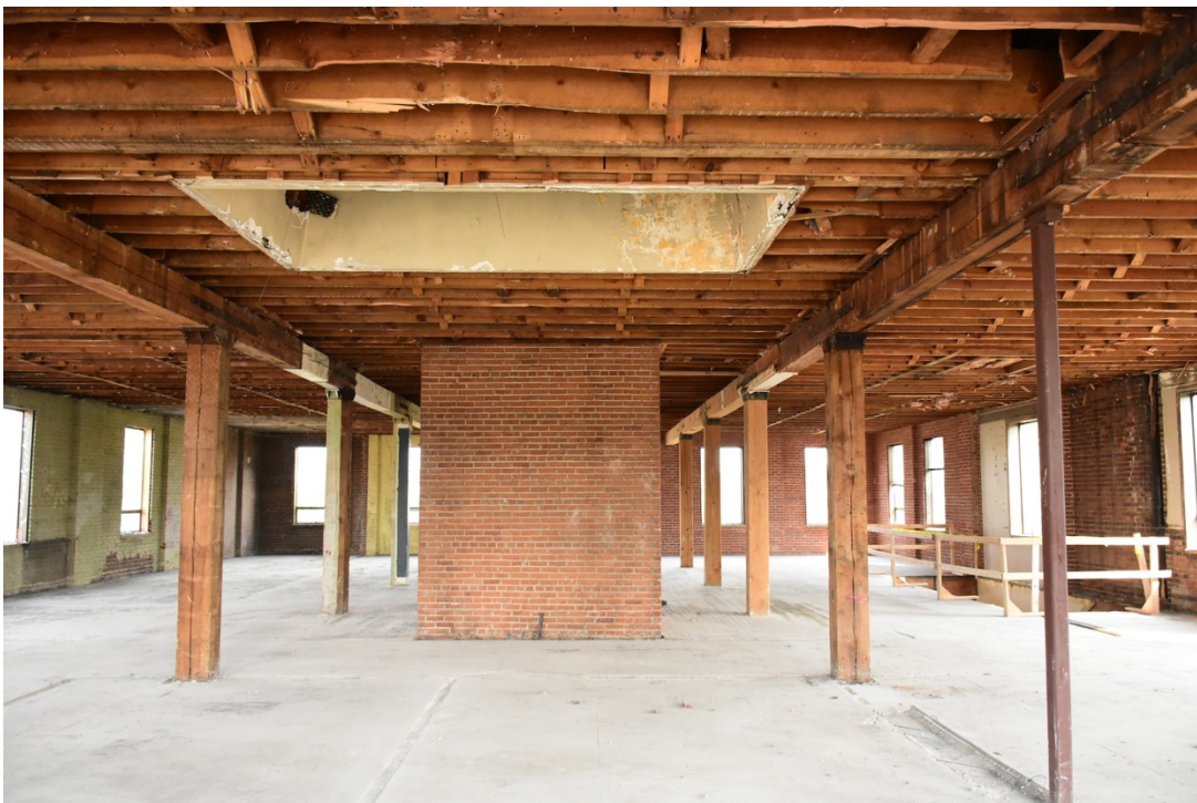
10. Second floor, looking north from south wall (skylight and elevator shaft)
