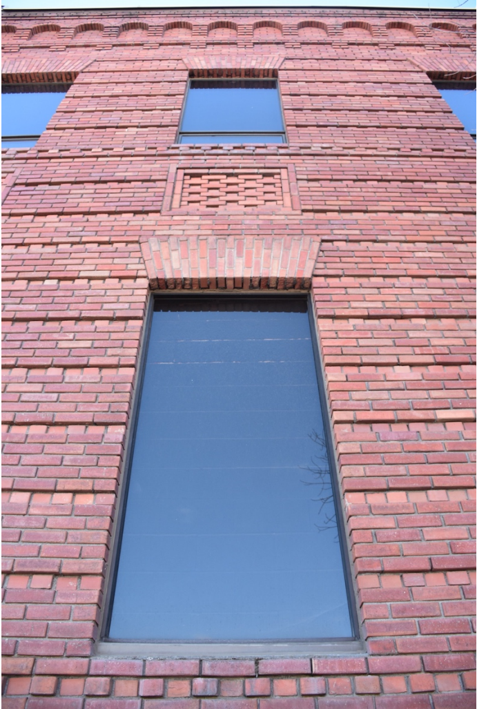
#12. Wall and parapet detail at southeast corner, looking west
