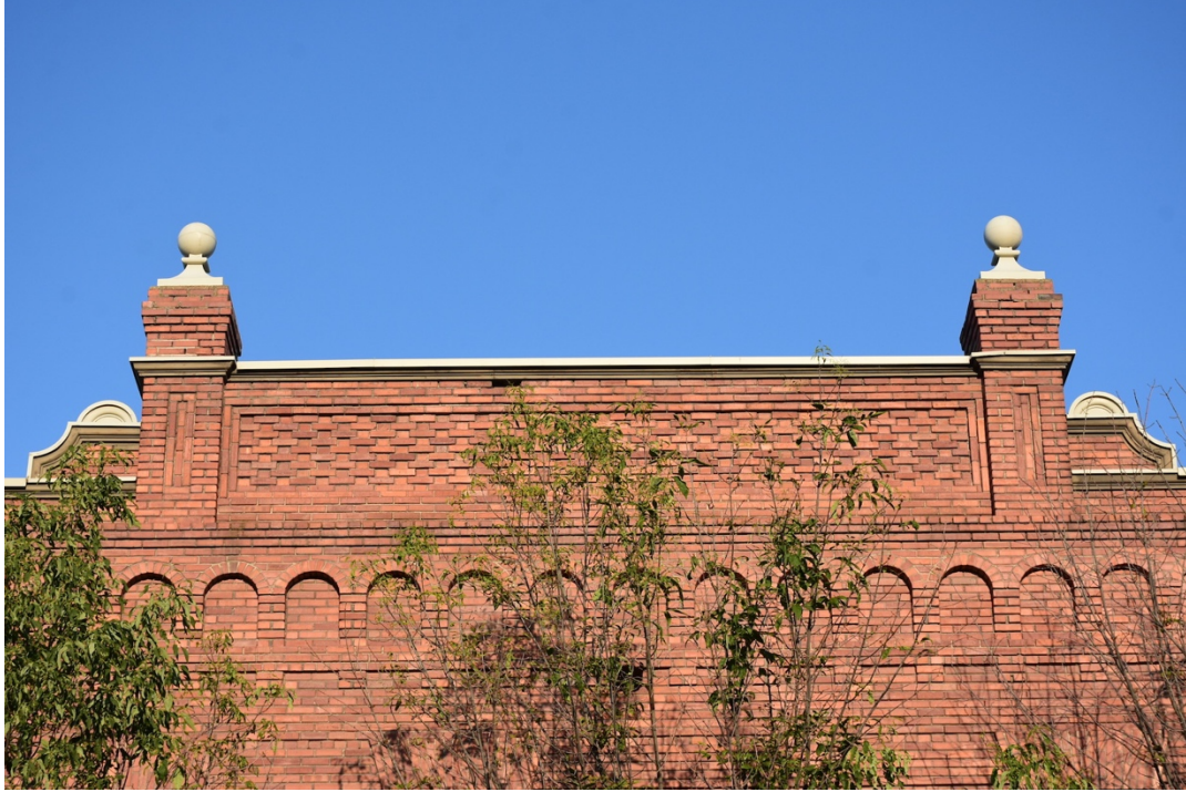
#9. Parapet terminating east facade, looking west
