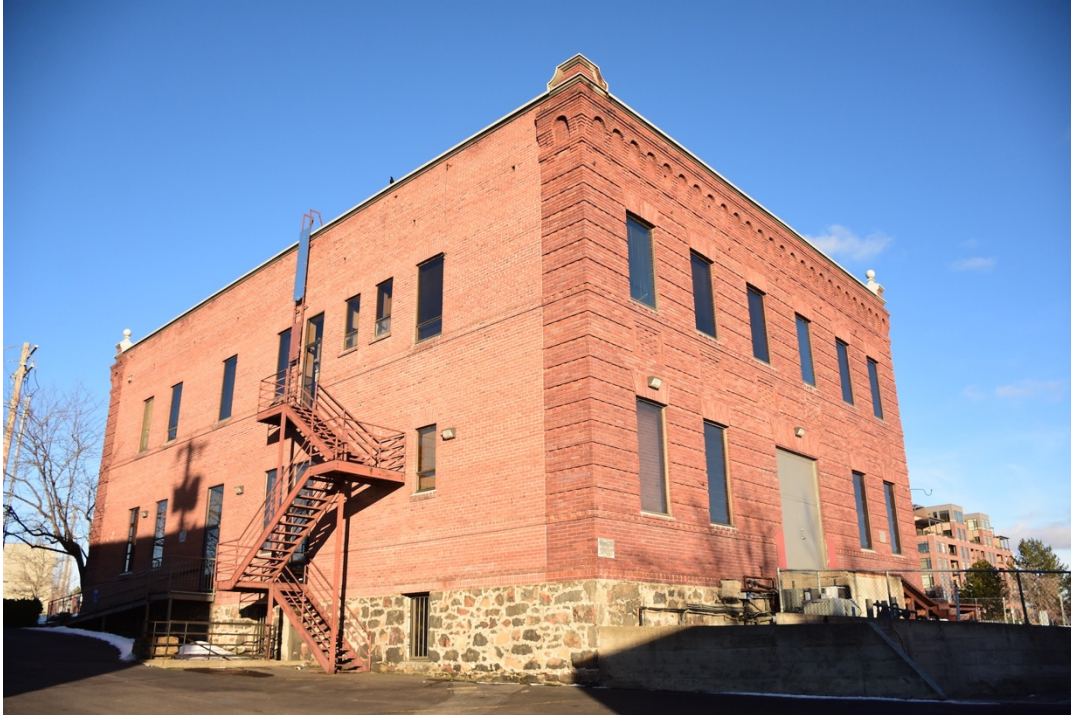
7. Southwest corner - south and west facades, looking northeast
