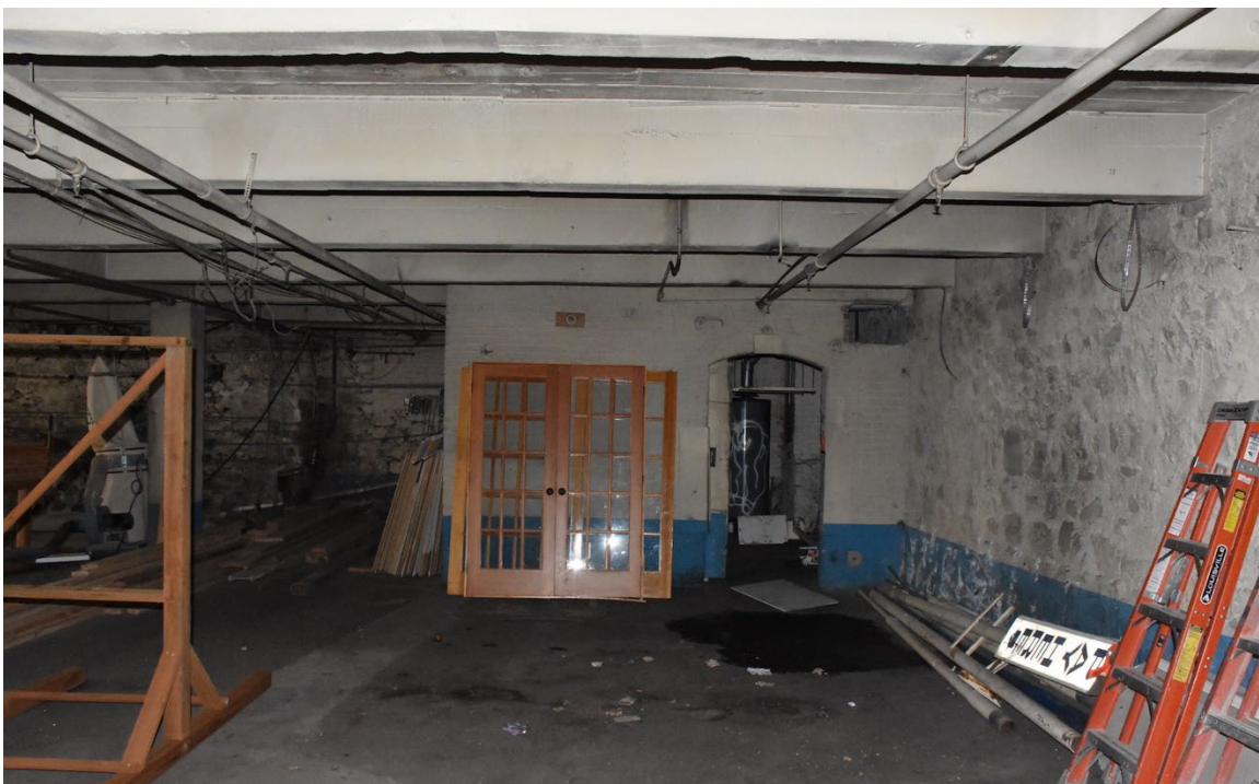
26. Basement - mechanical room in northeast corner, looking north
