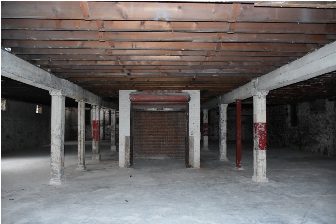
4. Basement - mid-section showing freight elevator, looking north
