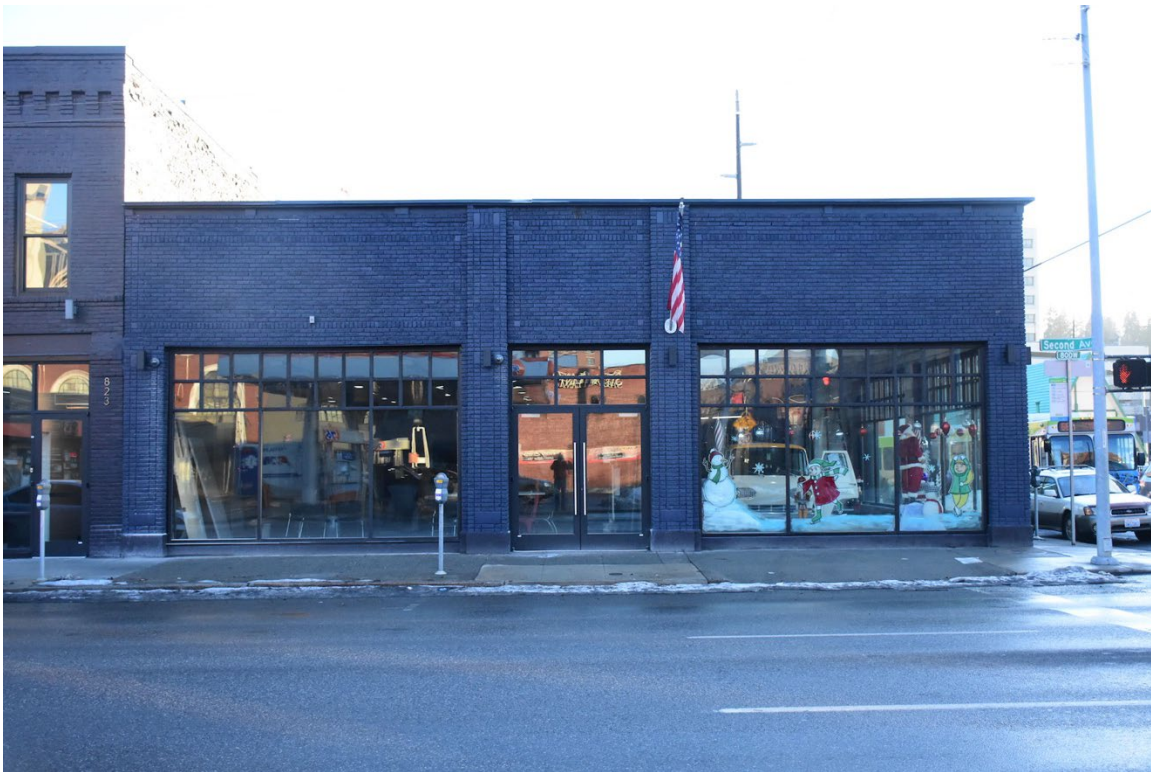
4. Front facade (north), looking south
