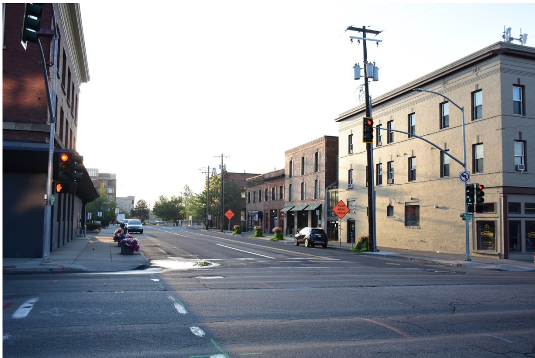
#2. Context along Broadway, looking east from Monroe Street
