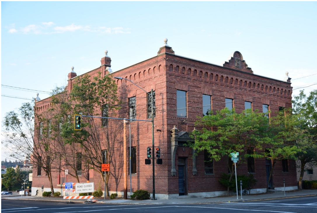
#4. Northeast corner - north and east facades, looking southwest
