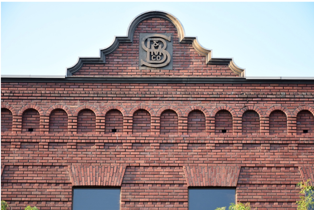
#8. Central pediment detail, looking south
