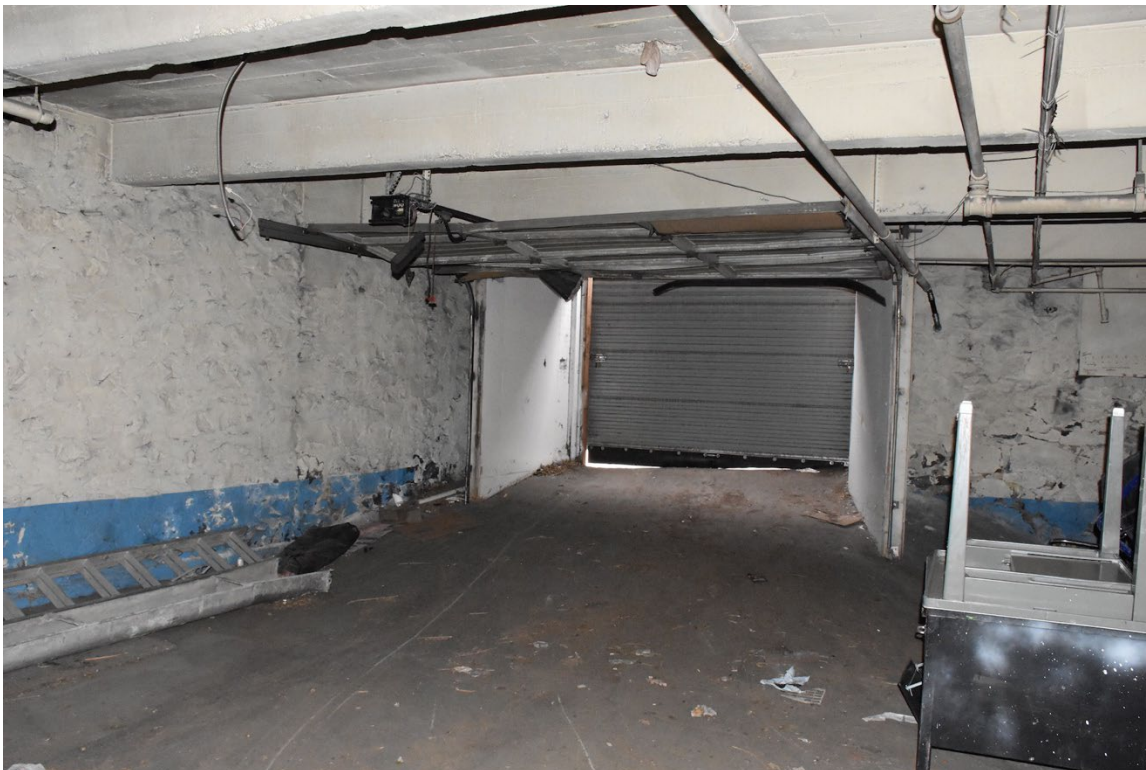
27. Basement - southeast corner garage door to alley, looking south
