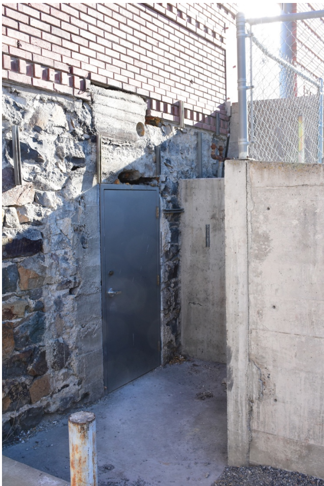
2. Entry to basement from south side.
