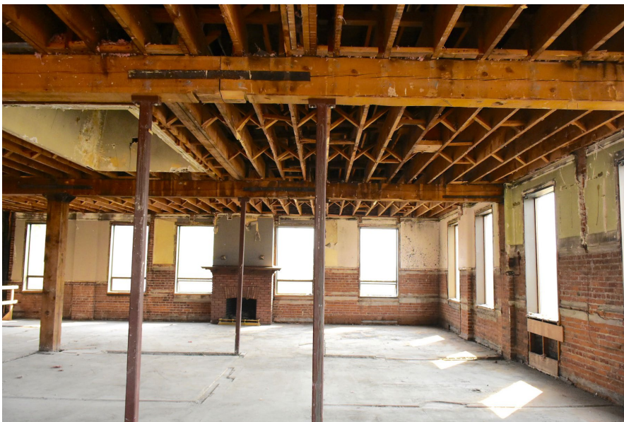
Figure 15: Second floor, looking east at the southeast corner and fireplace
