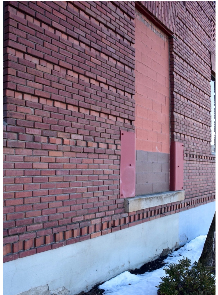
#14. Detail of east facade brickwork, looking southwest
