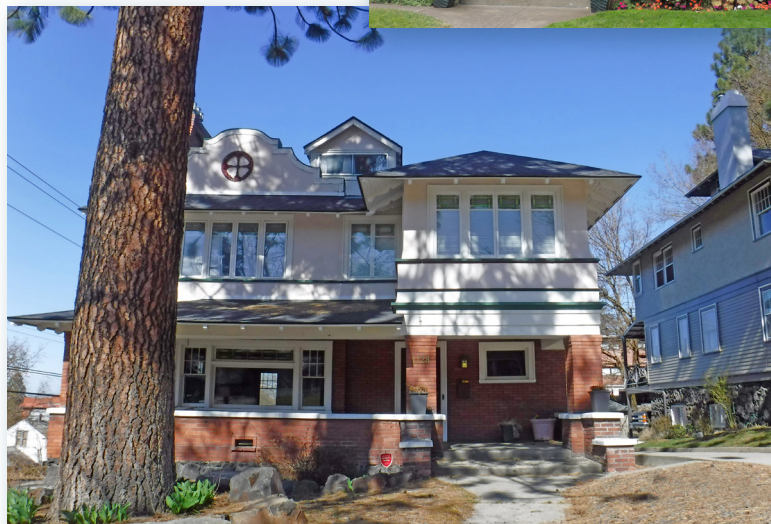
The house at 1128 W Eighth Avenue shows a hip roof, exposed eaves, and a mission style parapet.
