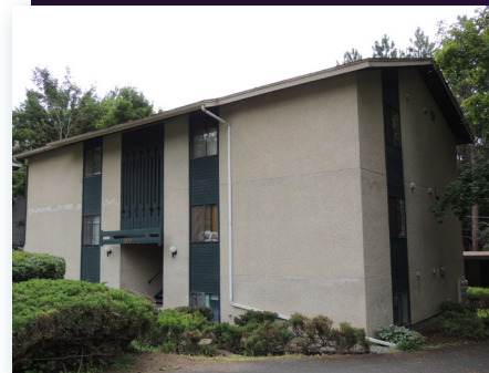
Vertical Plane Breaks at 909 W Thirteenth
