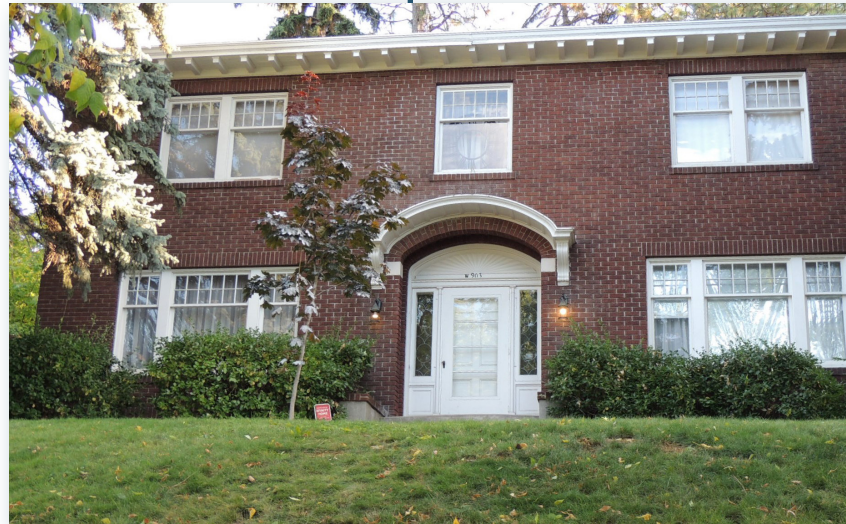
The Italian Renaissance style apartment building at 2306 W Pacific Avenue stands three stories tall in a rectangular plan that is capped with a flat roof edged with parapets exhibiting a dentilated cornice
