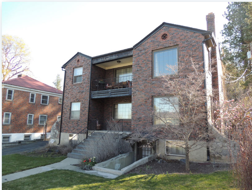
The small apartment building at 1023 S Monroe retains very good integrity except for the replacement of windows on the main facade. Right: The building in 1940, photo courtesy of the NWMAC L87-1.19183-40.
