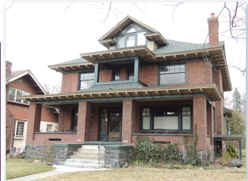
2927 S Adams Street: The full-width front porch is constructed with masonry columns and solid brick walls with drainage openings.
