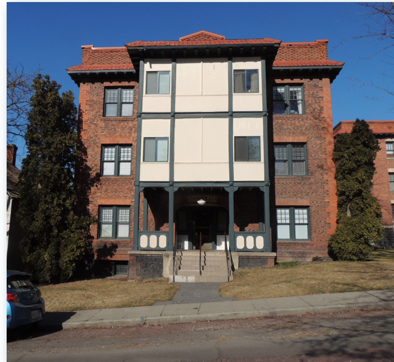
This multi-family apartment building at 1212 W Seventh originally had open or sleeping porches on the second and third floor. Although those features have been lost, the building still conveys its historic use and much of the original material remains.
