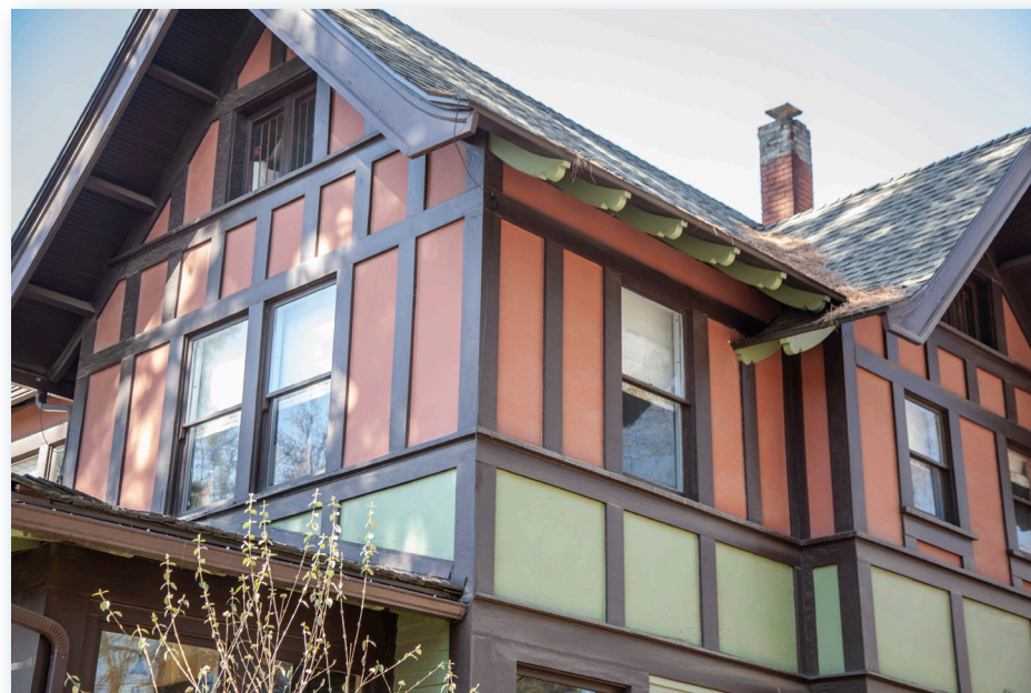
Original wood windows at the home at 1106 W Ninth Avenue.
