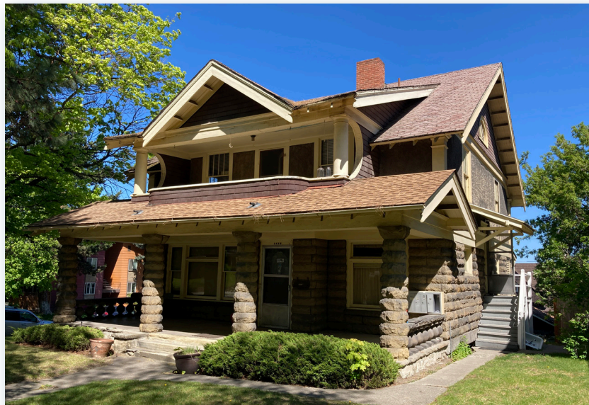
The house at 1432 W Seventh has interesting cut stone columns and first floor; a side gable front porch and deeply overhanging eaves with exposed rafter tails.
