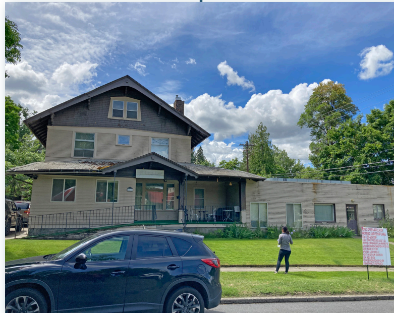
This house at 1117 W Tenth Avenue had a large, incompatible addition added in the 1950s when it functioned as a nursing facility.
