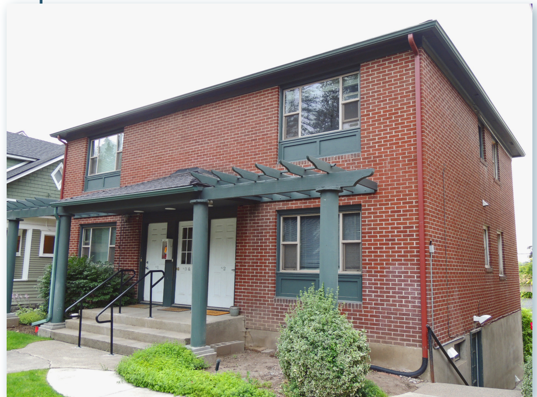
The small apartment building at 814 S Lincoln Place shows a tripartite window configuration.
