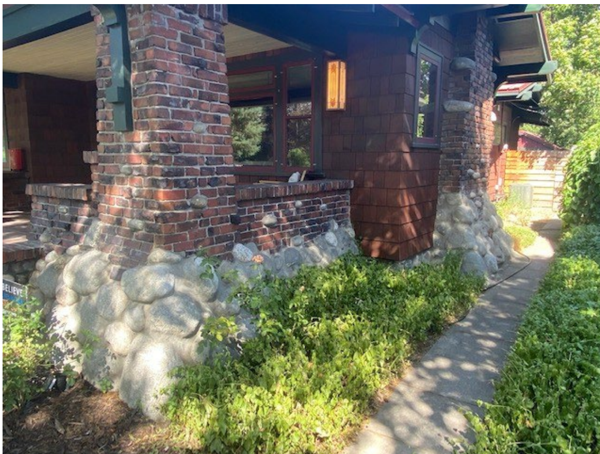
Picture 5: Detail of "peanut brittle" work with clinker brick, cobblestone
