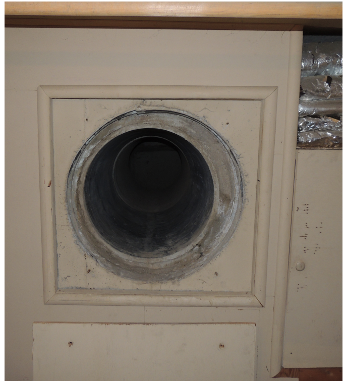
Fig. 12. Tunnel access point with plywood panel removed.
