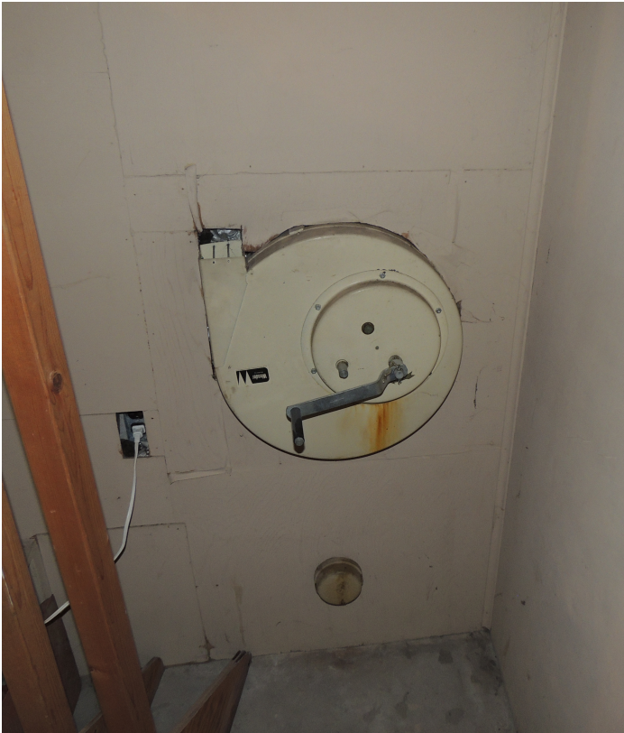
Fig. 11. Air blower in situ on the shelter wall with plumbing for toilet below it
