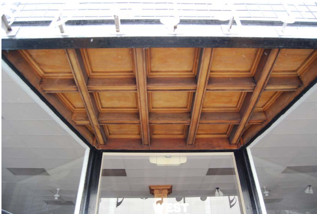
6. Coffered ceiling above main entry approach
