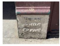
Figure 2. Cast iron pedestal detail showing factory stamp.
