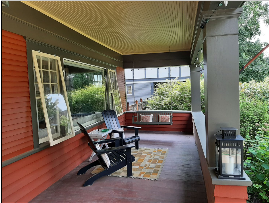
Photo 7 2024 photo of front porch, looking west
