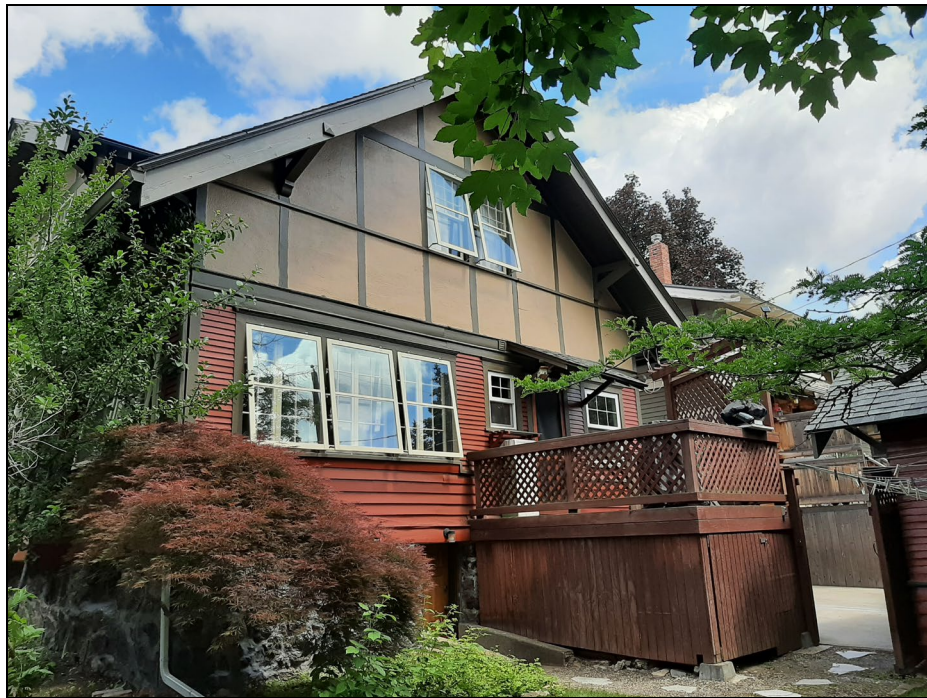
Photo 4 2024 photograph of south rear elevation of house
