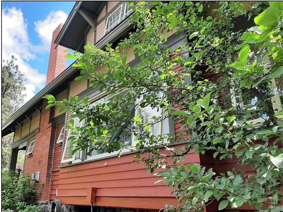
Photo 5 2024 photo of west elevation of the house
