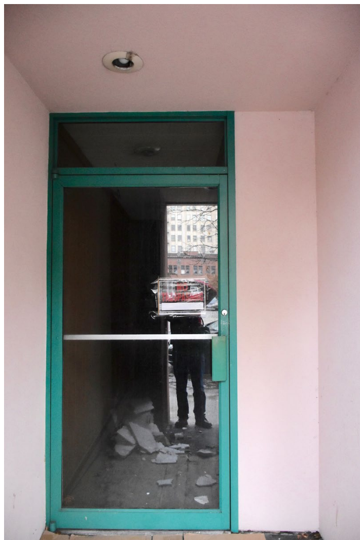
#12. Front entry door, looking south
