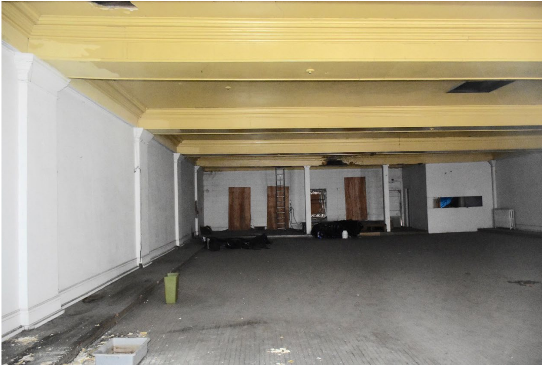
#25. Third floor - foyer, looking west from stair lobby along north wall
