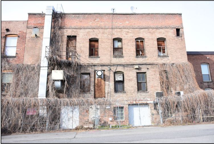
Figure 3: Rear elevation of the Wharton Building
