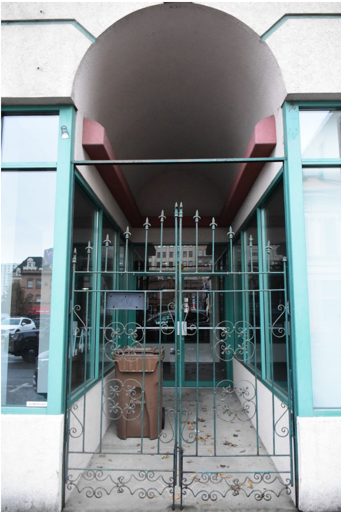
#1. Front Main Entry vestibule, looking south
