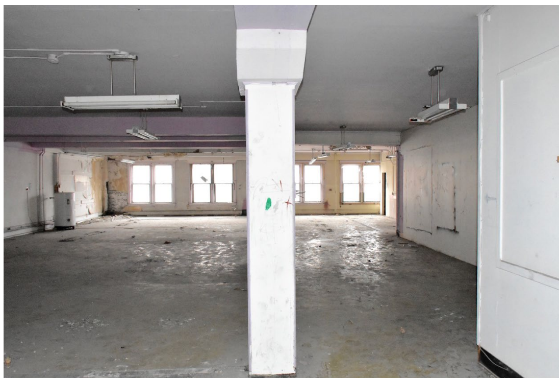
#17. Second floor - south room, looking west from room in southeast corner
