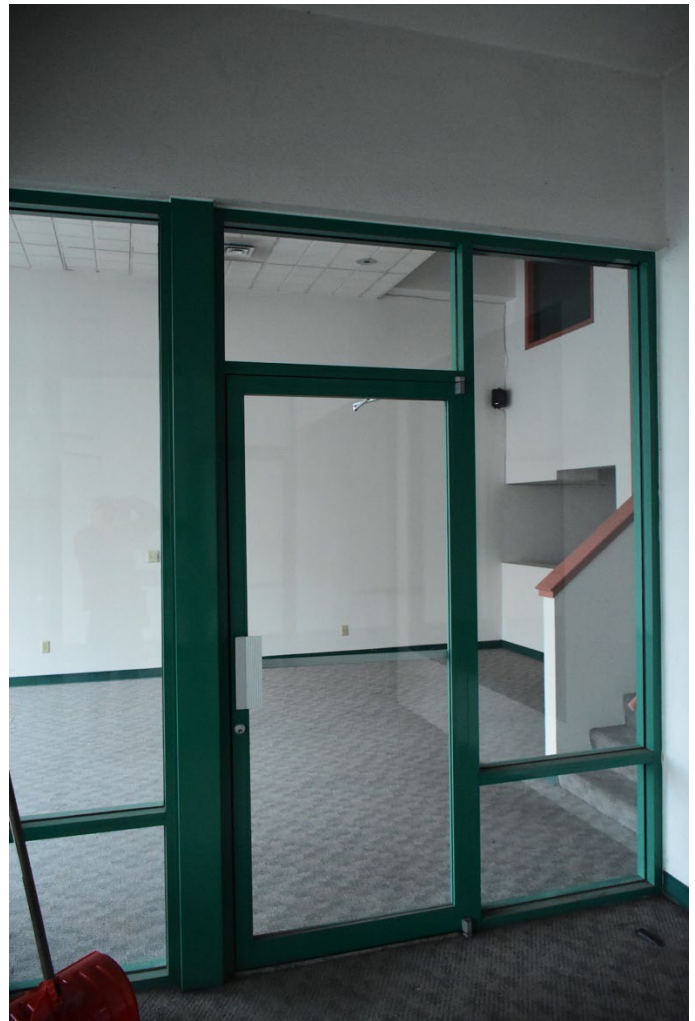
#2. Entry to reception area, looking east
