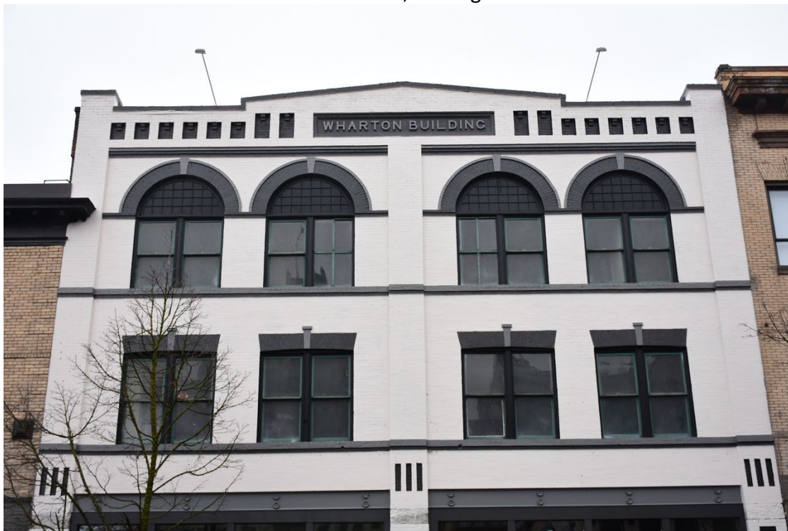
4. Front Facade, looking south
