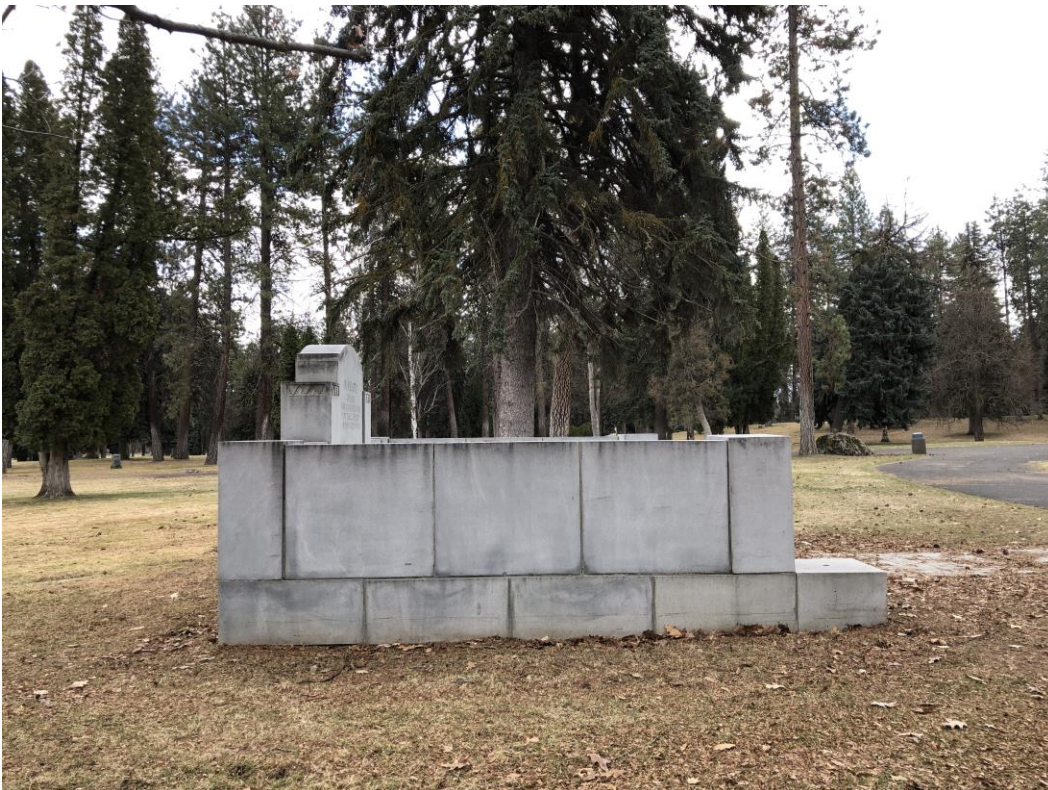
3 of 10. North side view of Cenotaph. - WA_SpokaneCounty_AmericanLegionCenotaph_0003
