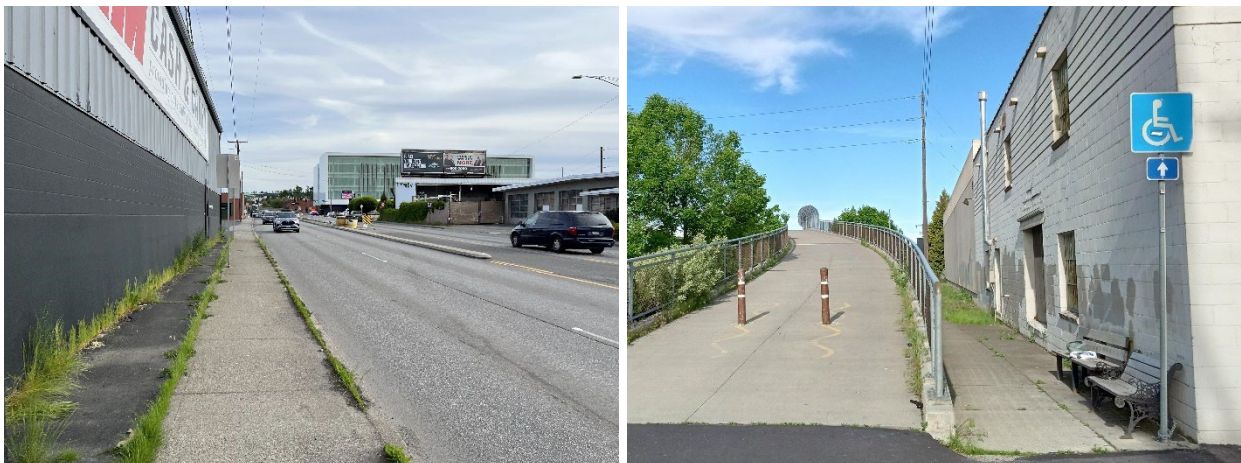
Figure 18. Left: A narrow sidewalk next to high-speed traffic on Hamilton St creates an unnerving walking environment. Right: The Centennial Trail bridge over Hamilton St is too steep to provide an ADA compliant pathway.
