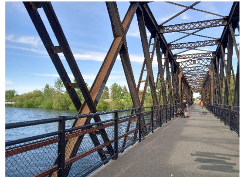
Figure 9. Iron Bridge walking/biking bridge
