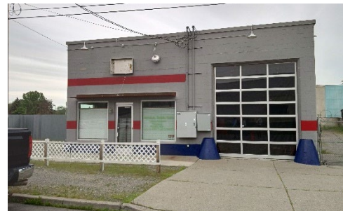
Figure 13. Vacant building in the industrial area.
