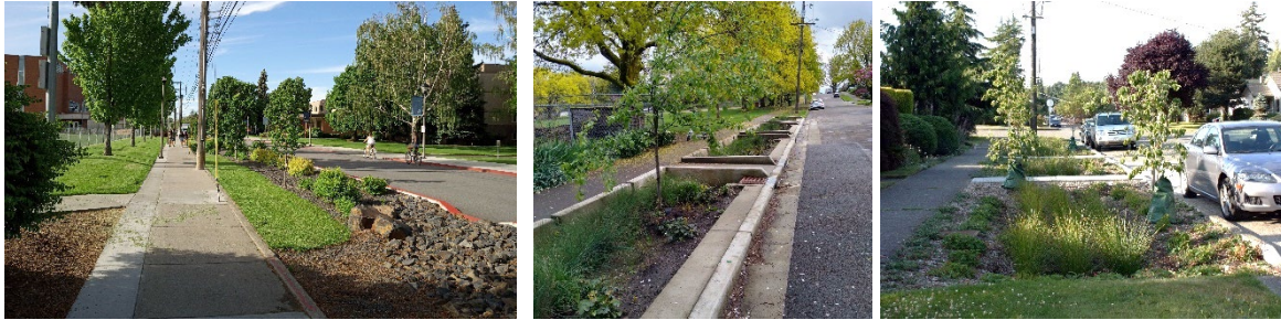
Figure 78. Examples of GSI streetscape improvements.
